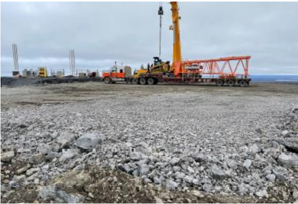
Extended Crane Pad Area
