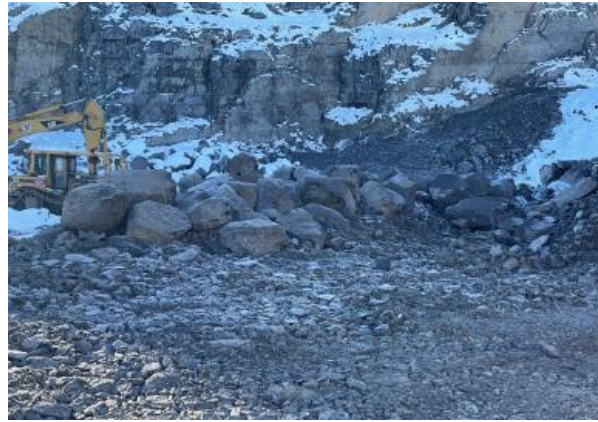
Oversized Material Removed from Blast Rock
