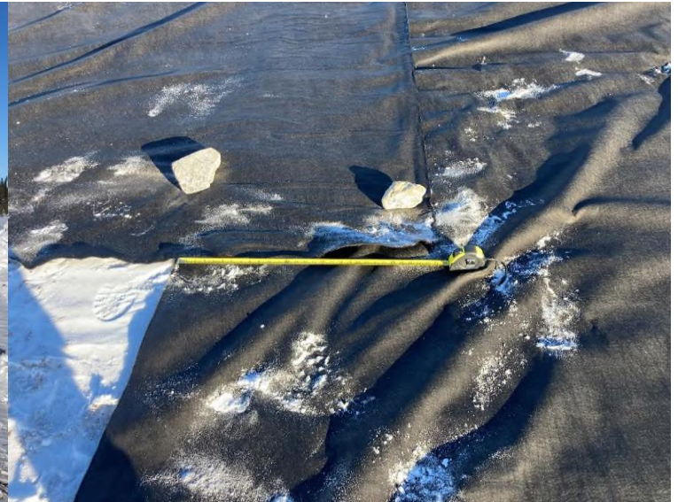
Checking Geotextile Overlap
