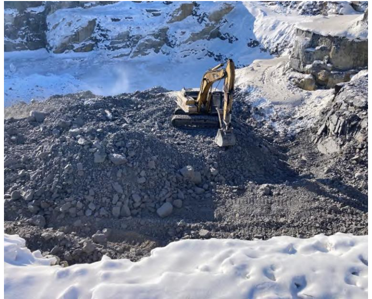
Excavator Pulling Blast Rock
