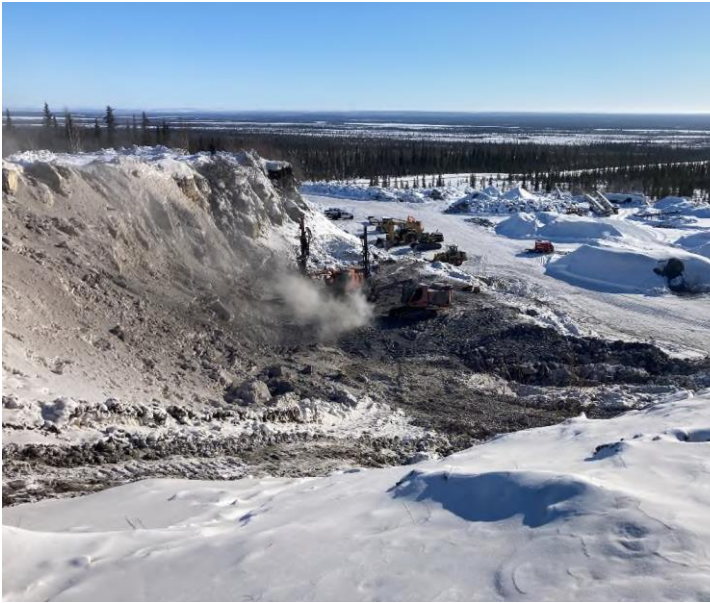
Two drills at Blast Area #2
