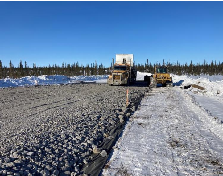
Truck Offloading at Access Road
