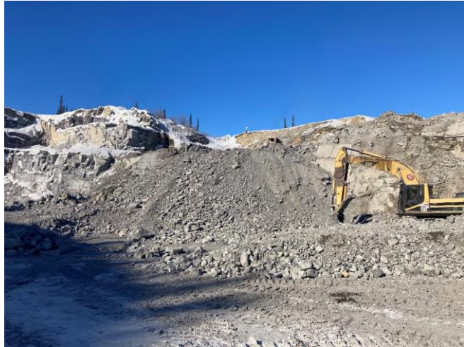
Blast #1 Stockpile Development
