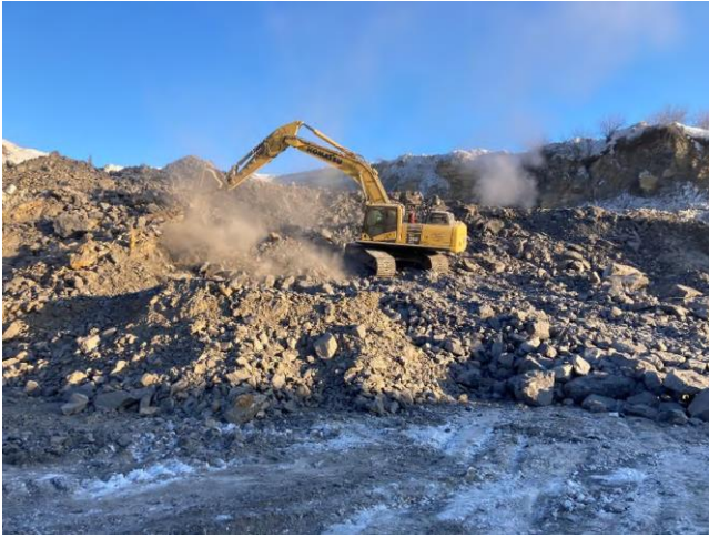
Clearing Blast #2 Stockpile
