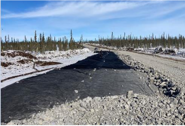
Geotextile Placement
