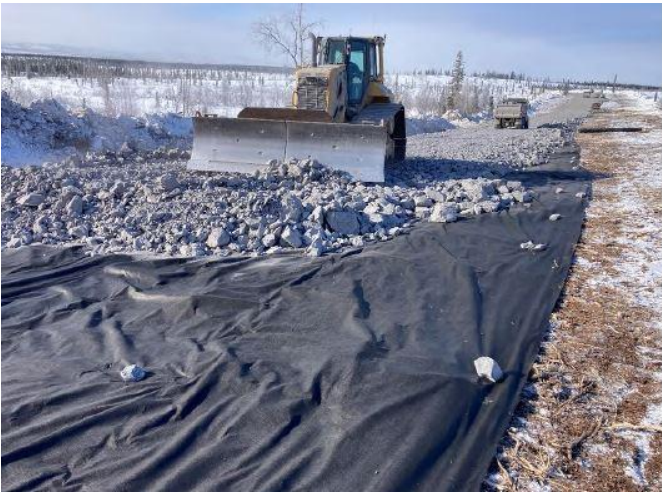
Dozer Spreading Rock
