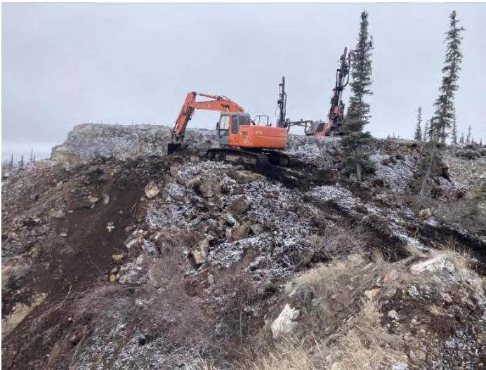
Removing Overburden
