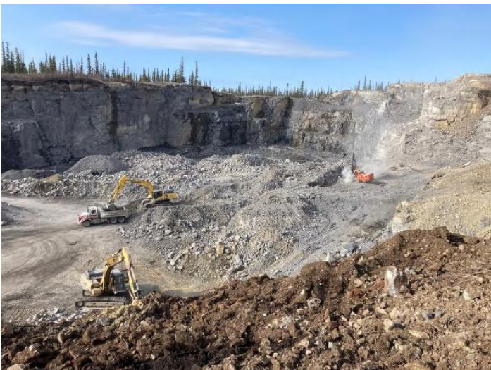
Loading/Drilling in Quarry
