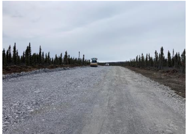
Compacting Ahead of Second Lift
