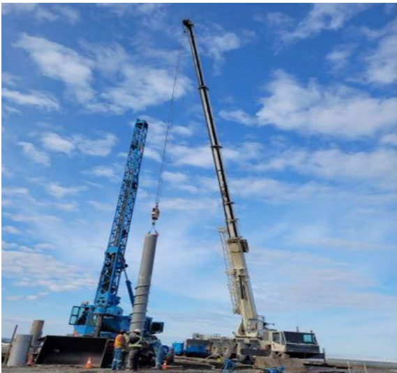
Placing Pile
