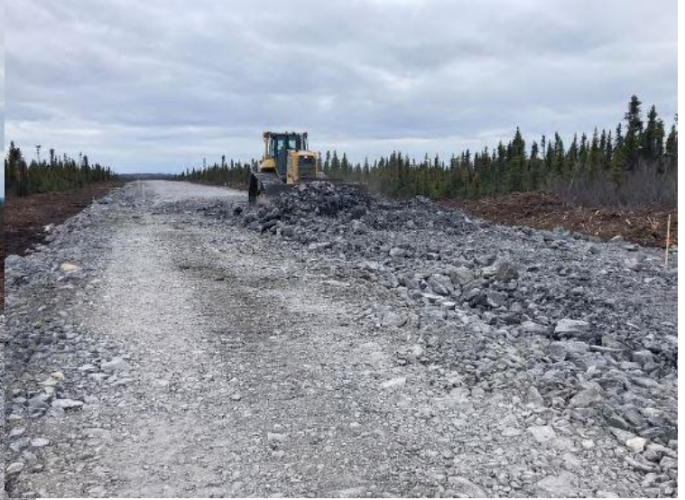
Placing Second Lift
