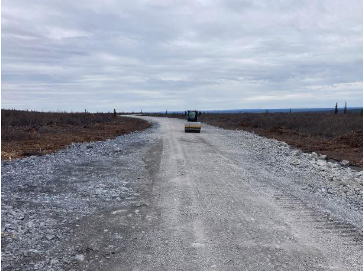
Compacting First Lift
