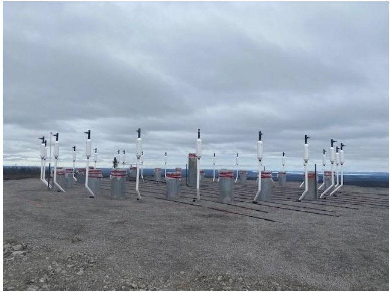
Horizontal Thermosyphons
