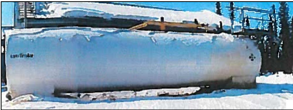
Figure 3 – Diesel fuel tank.
