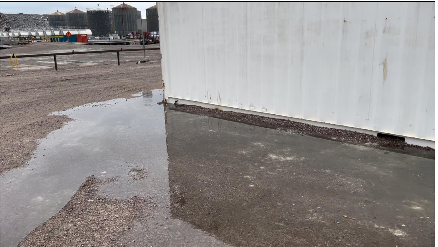
Figure 2. Spill at Dorm A11 Lift Station, GNWT Spill #2024259
