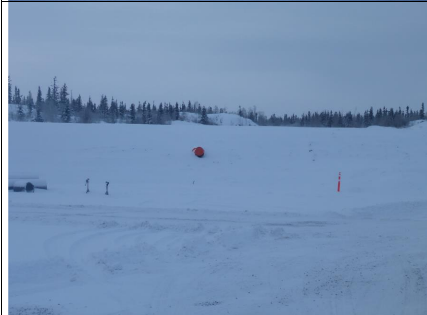
Photo #3: Overview of the non-hazardous landfill
