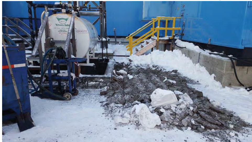
iv) Follow-up : Excavated soil to determine extent of spill
