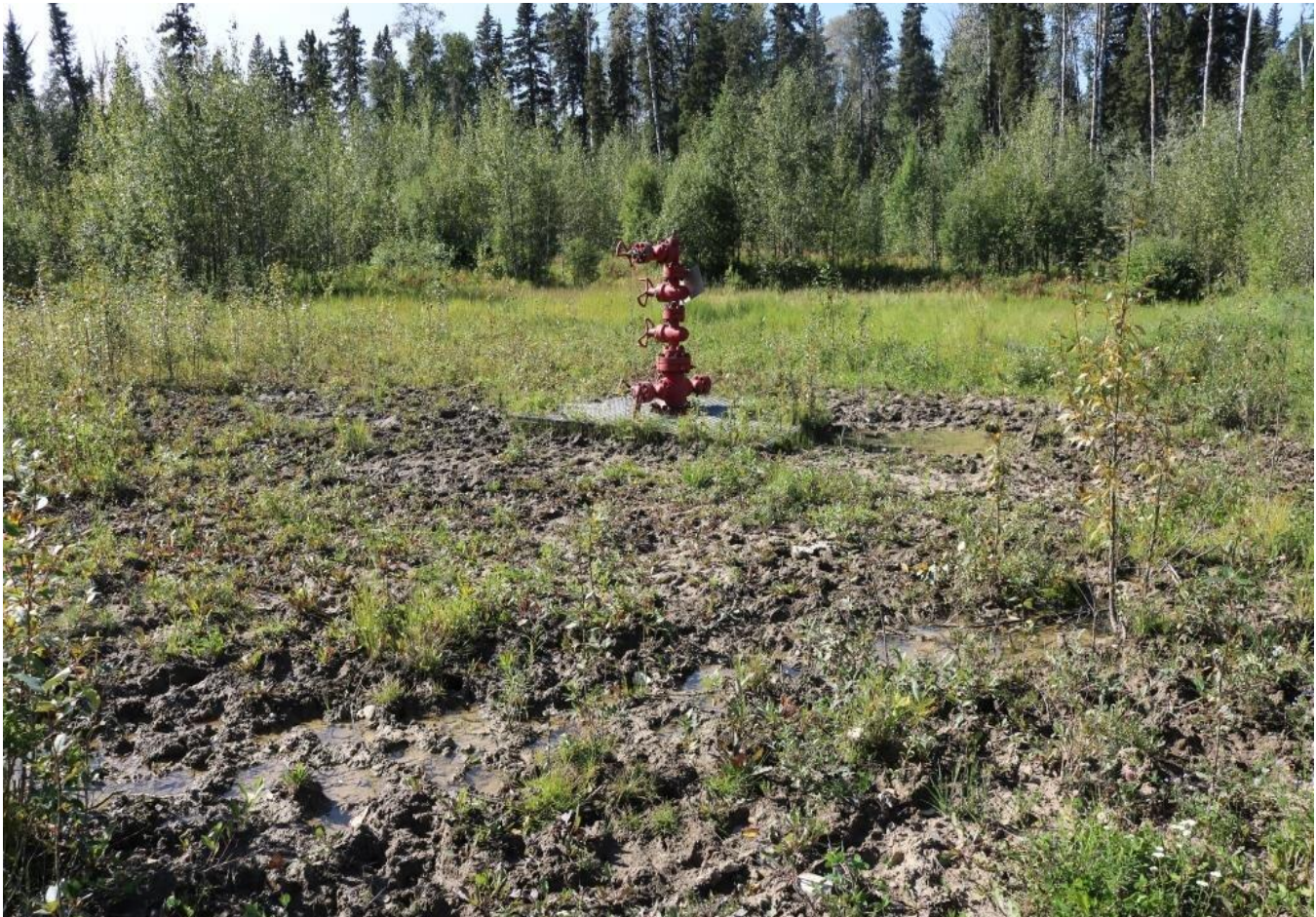
Bare ground around I-02 wellhead
