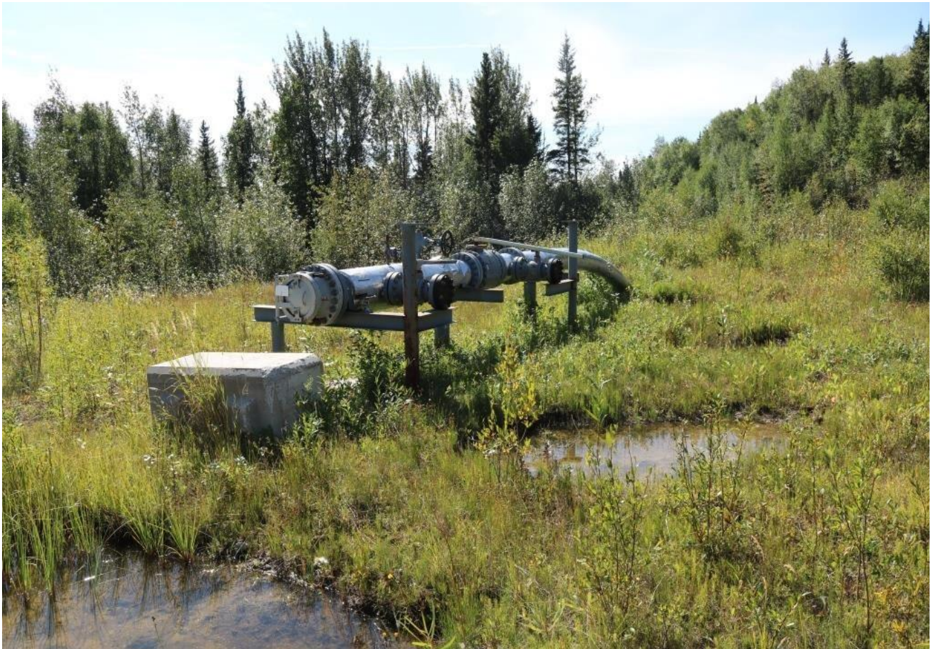
Riser on F-36 well site
