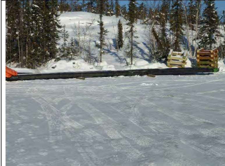
Photo #6: Piping staged for the competition of the project.
