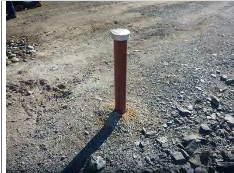
Photo #1: Overview of drilling location D21C-S019-18
