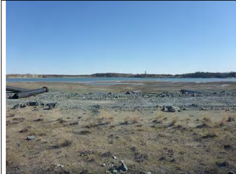
Photo #2: Overview of the Northwest Pond looking Northeast
