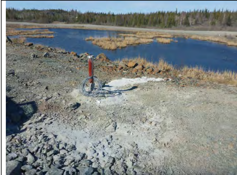
Photo #3: Overview of drilling location D21D-S019-13. Note the drill cuttings left after the demobilization from site.
