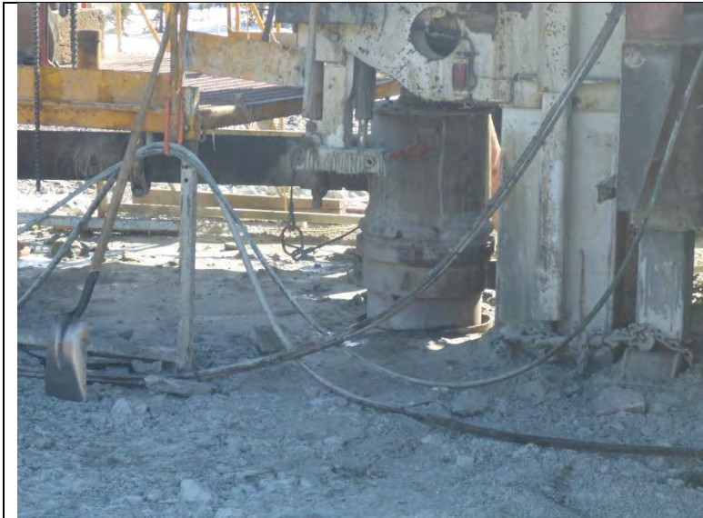
Photo #5: Close up of the drilling rig.
