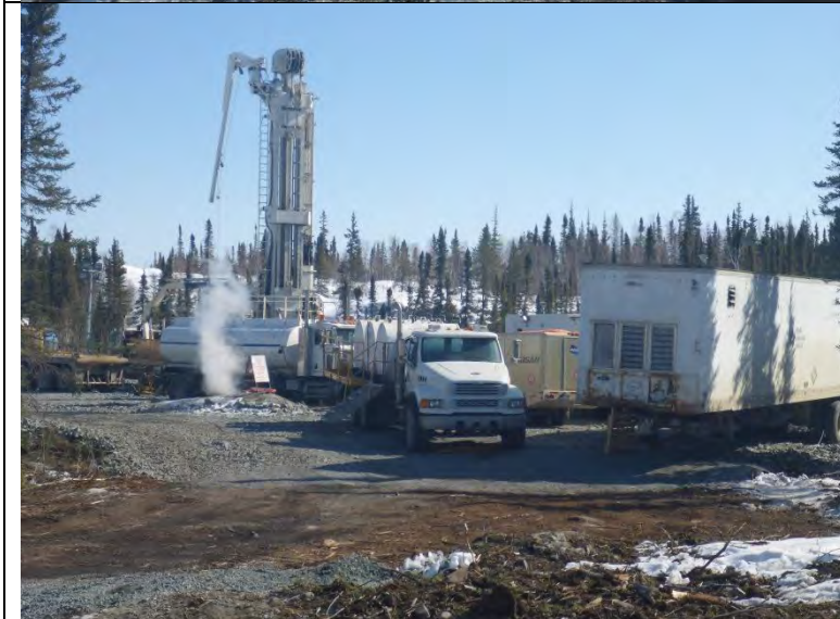
Photo #3: Overview of the drilling operation.
