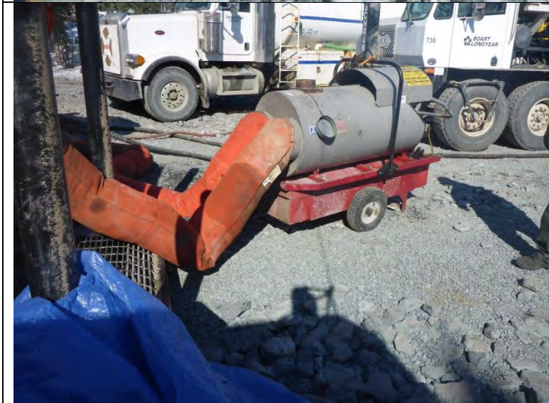
Photo #8: Frost fighter without secondary containment.
