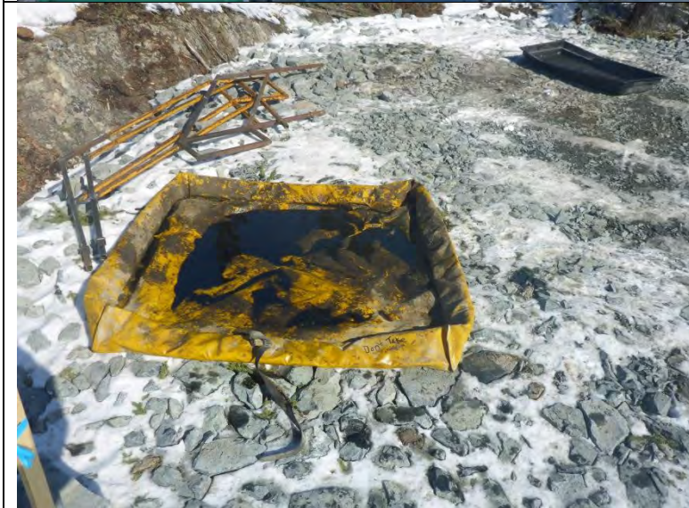
Photo #7: Drip tray containing waste oil. Note that some of this oil had spilled over to the surrounding environment.
