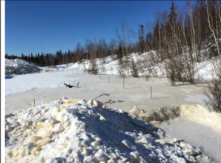
Photo #11: Posts that remain encapsulated in ice at the Bullmoose creek.
