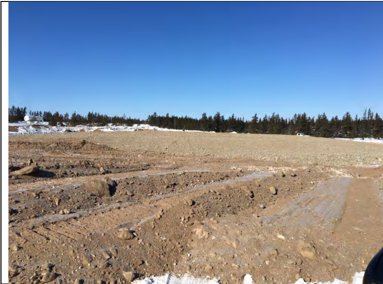
Photo #9: Bullmoose landfill in final stages.
