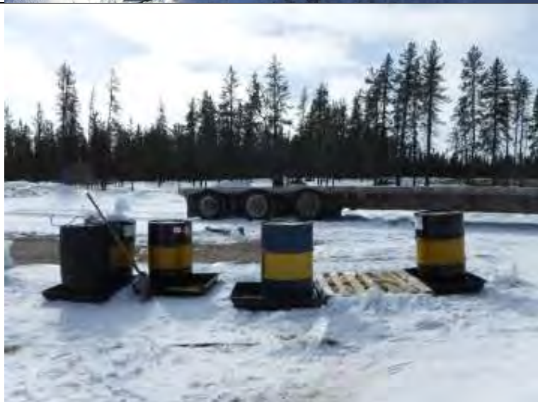
Photo #15: Secondary containment for fuel drums mitigated post inspection.
