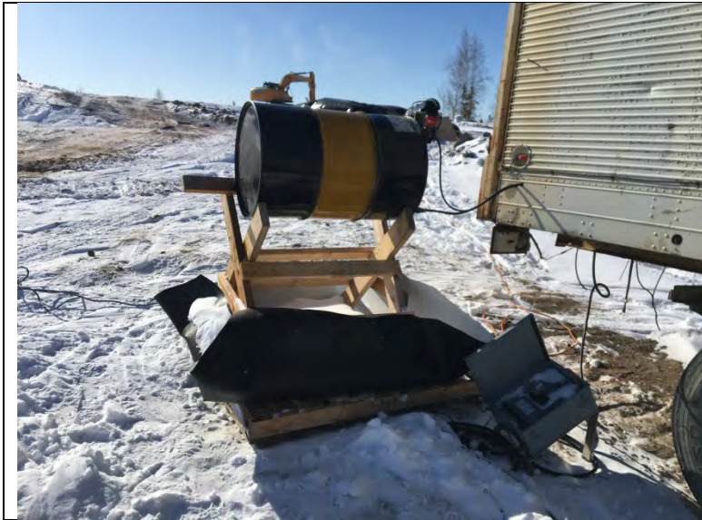
Photo #5: Fuel drum for parts van at Alimak does not have adequate secondary containment.
