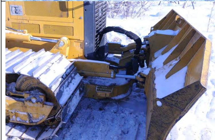
Photo #7. Close up of Dozer in Picture # 6.
