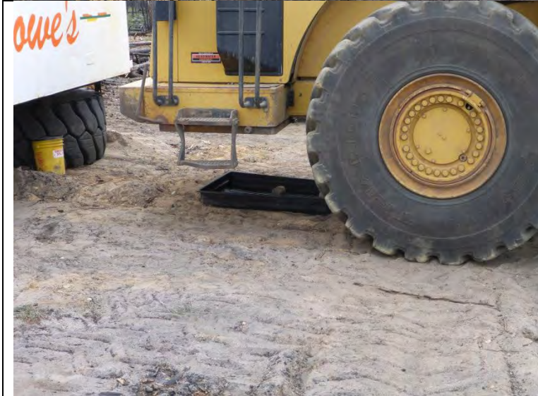
Photo #3: Drip tray placed underneath stationary vehicle.
