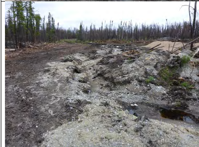
Photo #7: Trench dug at Beaulieu Site to facilitate dewatering.
