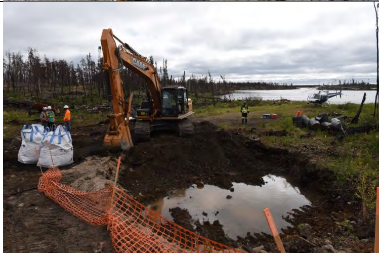
Photo #10: Clean up contaminated soil at Spectrum site.
