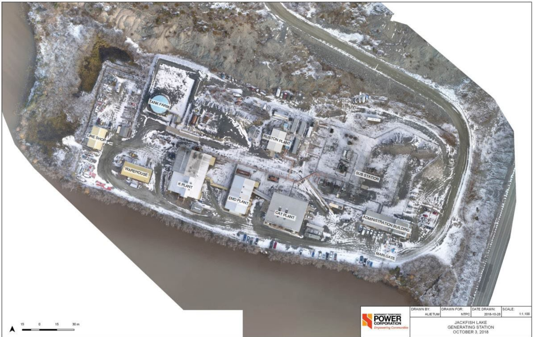
Figure 1-2 Jackfish Lake Generating Station
