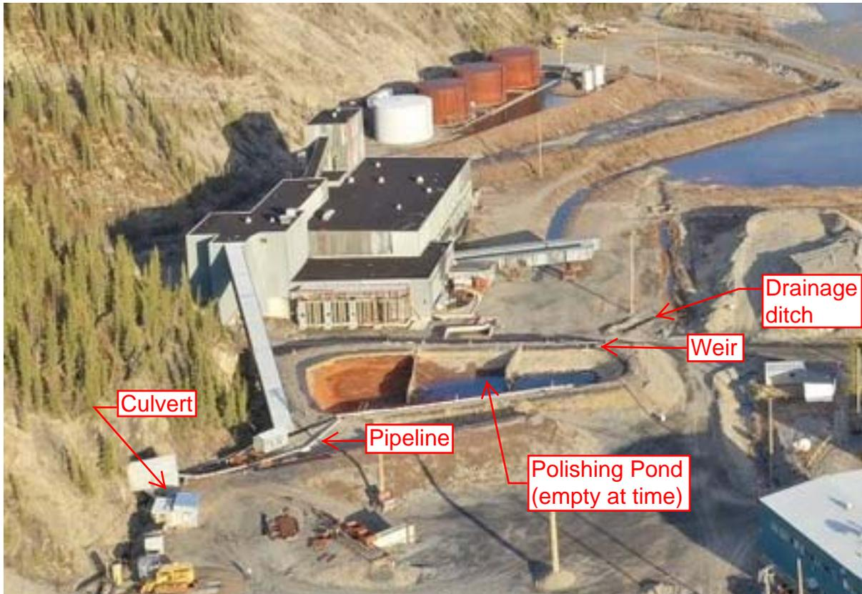
Site surface water runoff collects in pre-existing ditches which drain to the Catchment Pond. There, surface water co-mingles with treated mine water before discharge to Harrison Creek via a culvert which has a gate weir control point.
