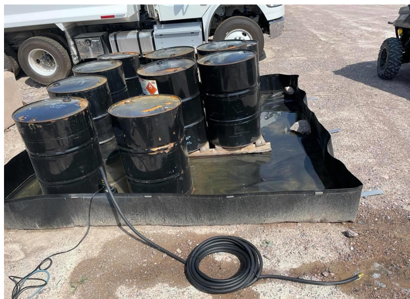
Figure 2 - Portable secondary containment under multiple drums
