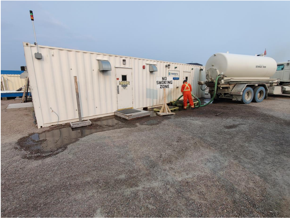
Figure 3. Photo of ongoing clean-up of GNWT Spill #2021309
