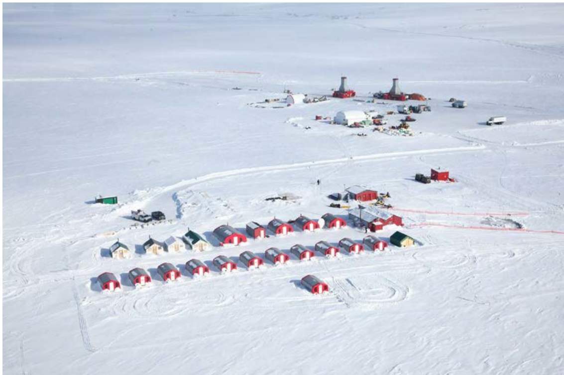
Figure 4: Aerial photos of Bob Camp (upper picture) and Kelvin Camp (lower picture) (2015)
