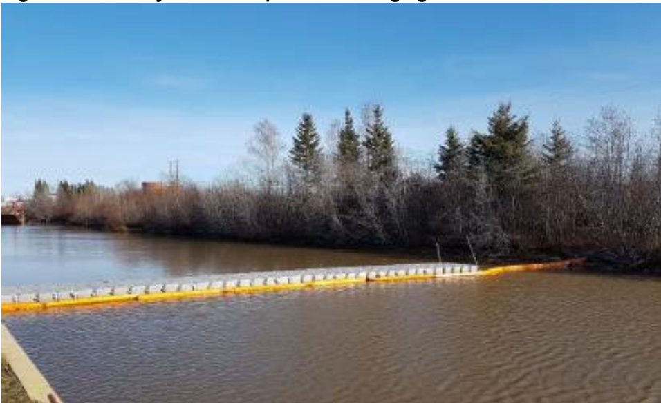
Figure 1- Turbidity curtain in place for dredging
