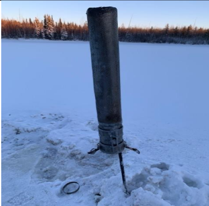
Photo 1. Water pump fish screen located at the little lake.
