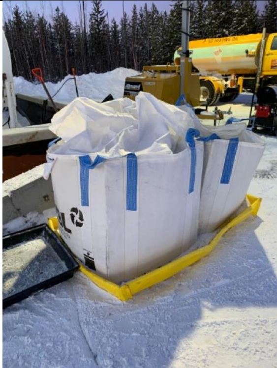
Photo 5. Contaminated snow ready for shipment with drip tray underneath
