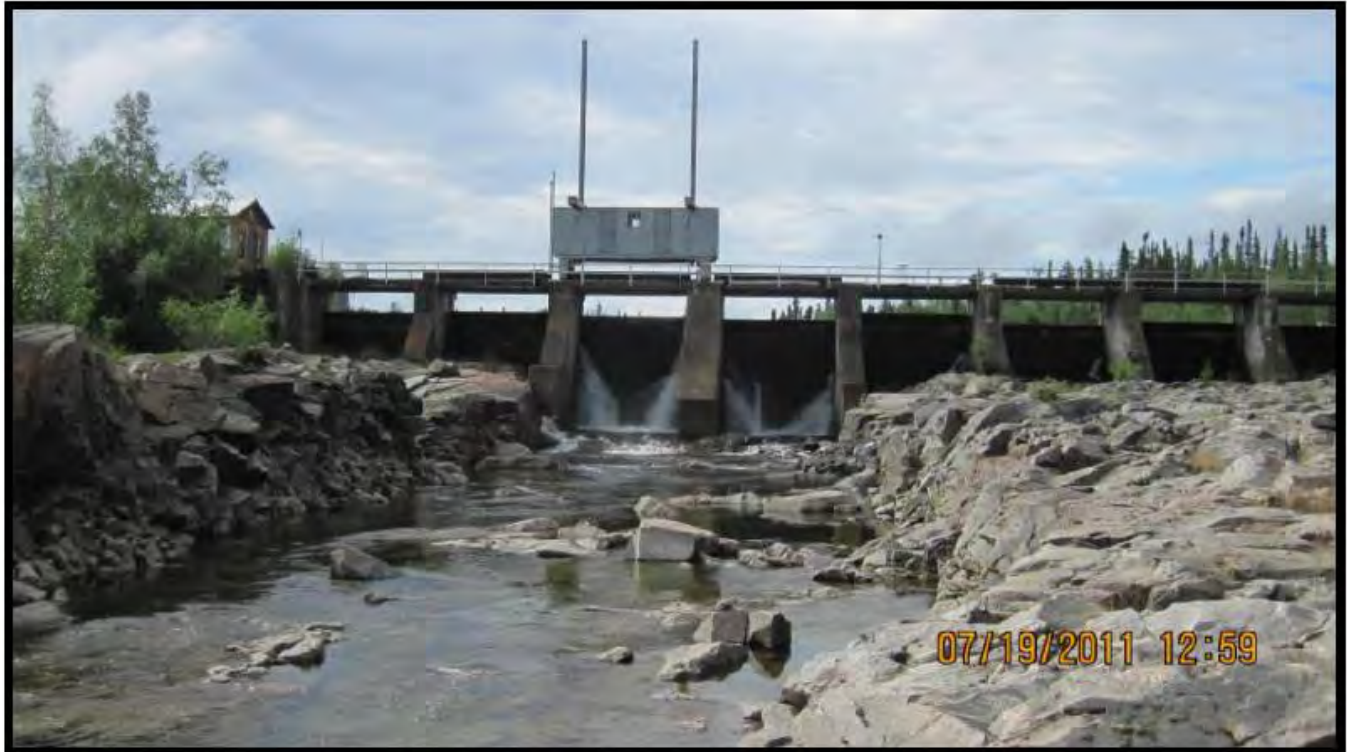
Figure 1: Snare Rapids – Spillway 5B: View from Downstream
