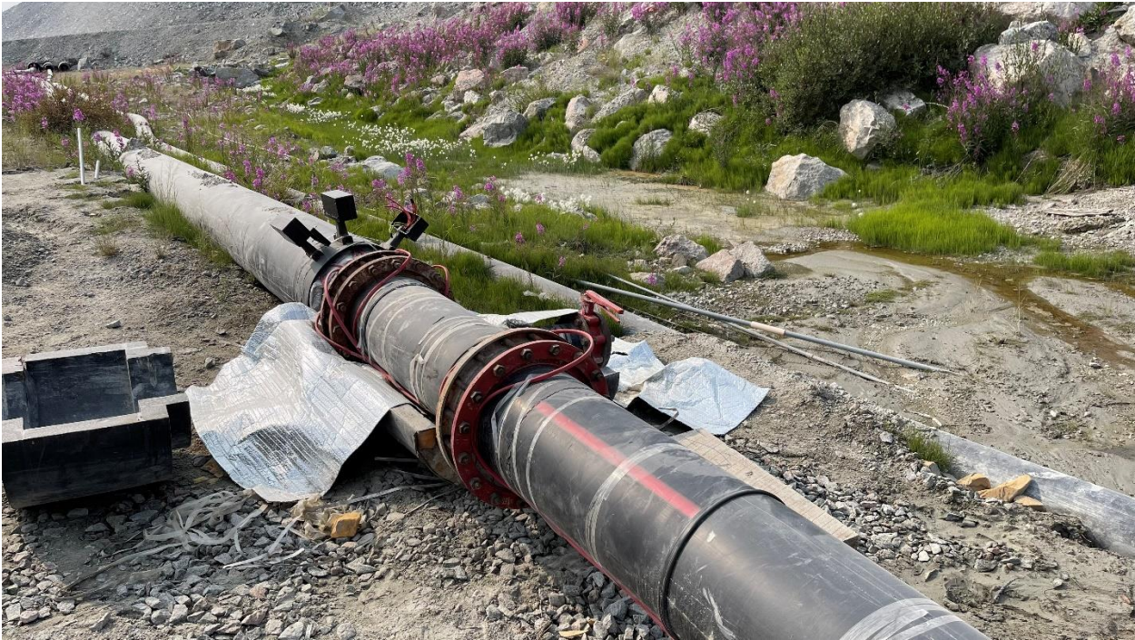
Figure 4: Repaired section of pipeline
