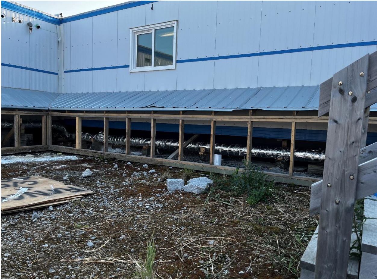
Figure 4: Inspected and repaired pipe section
