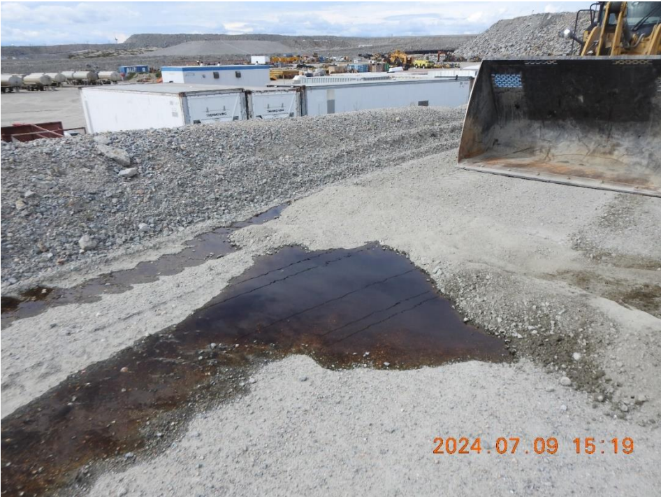
Figure 5: Rapid construction of gravel berm to limit downhill flow of spill
