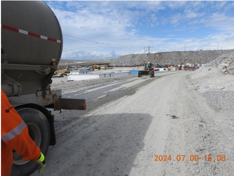
Figure 2: Location of spill on hill leading out of the Metcon Yard
