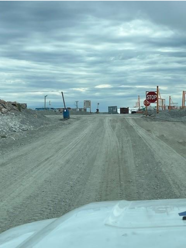
Figure 6: Spill area post-clean up
