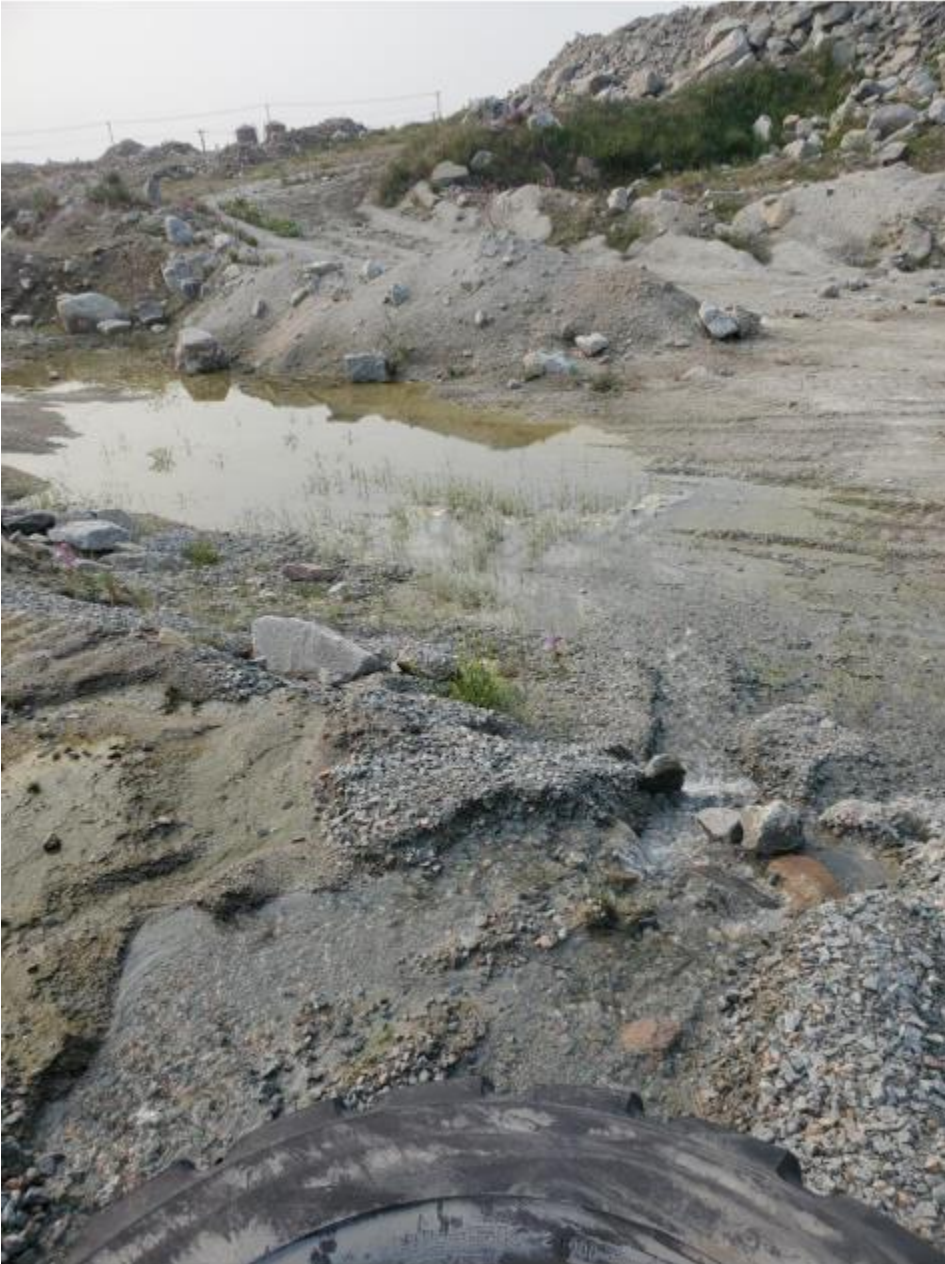
Figure 2: Spilled material exiting berm and pooling.
