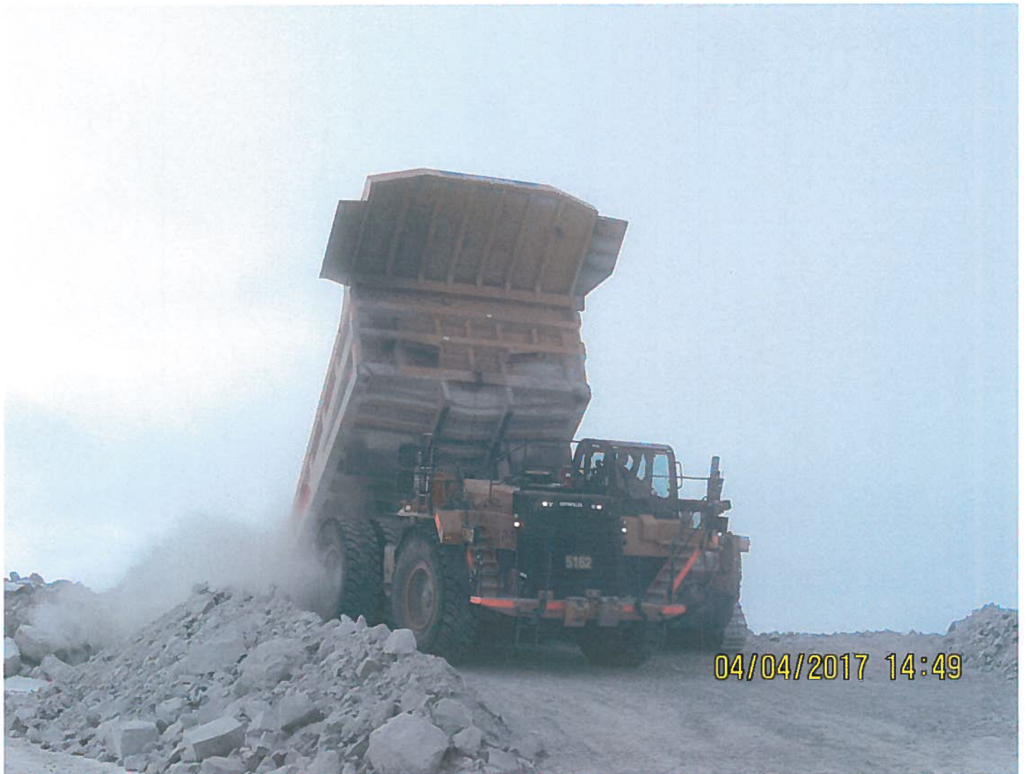
Photo 3: Sable Crusher Pad - Clean granite from the Sable Quarry is loaded into haul trucks and stock piled near the crusher pad.
