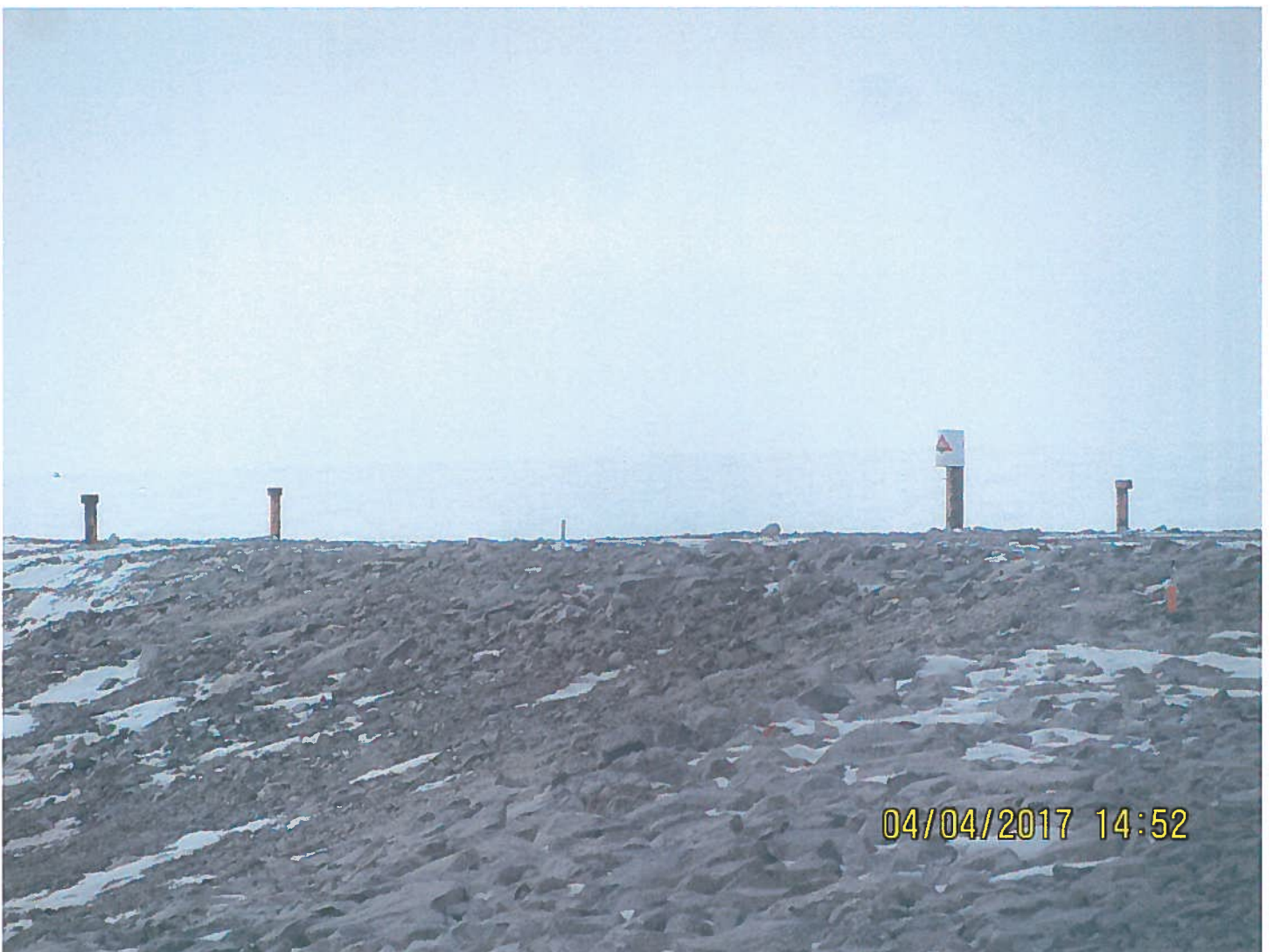
Photo 6: Two Rock Frozen Core Dam - A total of 9 vertical ground temperature monitors were installed within the Two Rock Frozen Core Dam to a depth of approximately 8-10 meters
