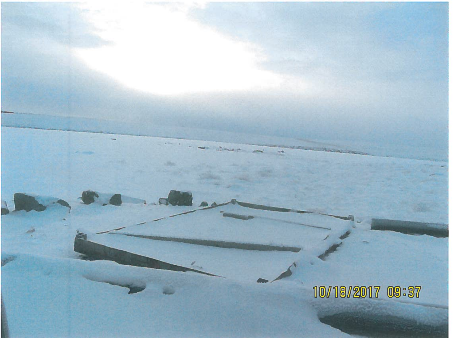
Photo 6: Two Rock Sedimentation Pond - The water pump that was installed in this containment tray on the west side of Two Rock Sedimentation Pond has now been removed.
