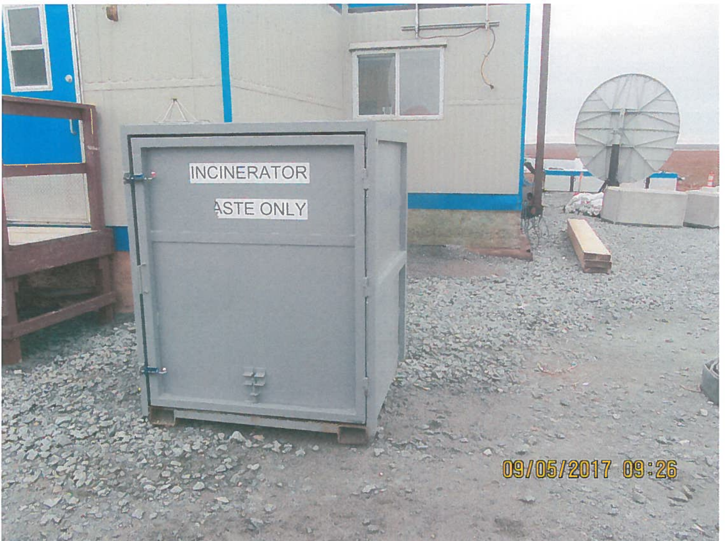
Photo 6: Sable Office Complex - All garbage that requires incineration is stored in a secure bin. Garbage is removed to the Incinerator building on a regular basis.
