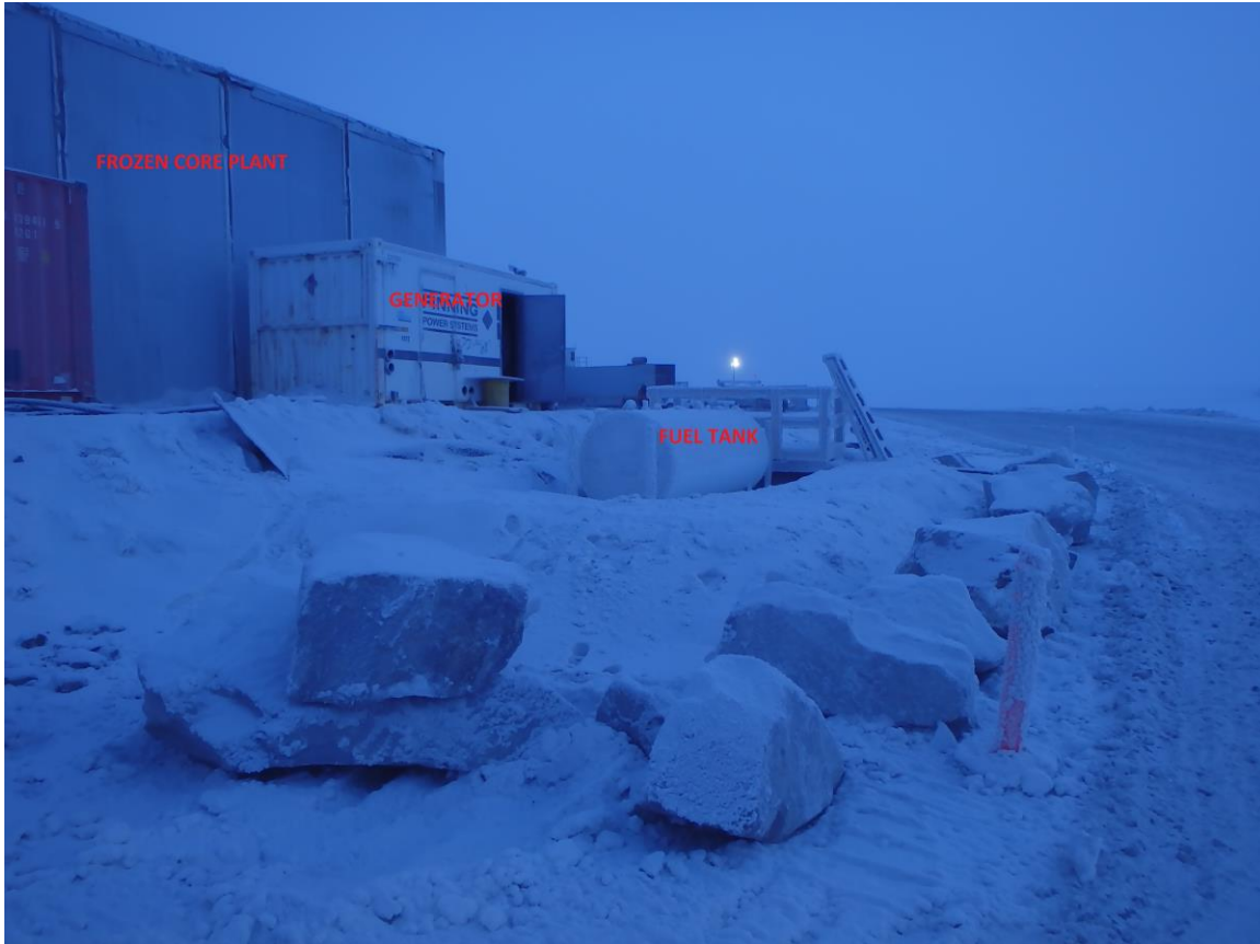
Attachment 2: Photograph of 4500 L fuel tank in lined containment berm
