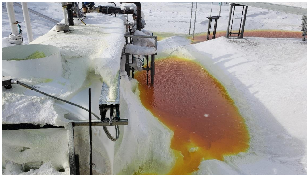
Figure 2. Pooled Diesel near Generator Day Tank (March 21, 2019)
