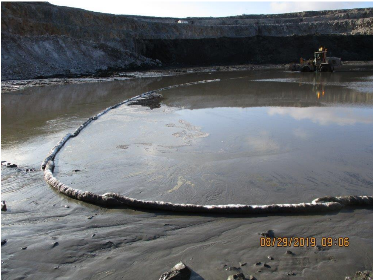
Figure 2. Spill booms used to coral hydraulic oil within Sable Pit
