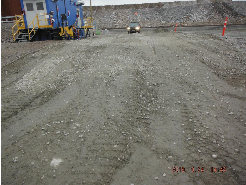
Figure 2. Lined pad after clean-up
