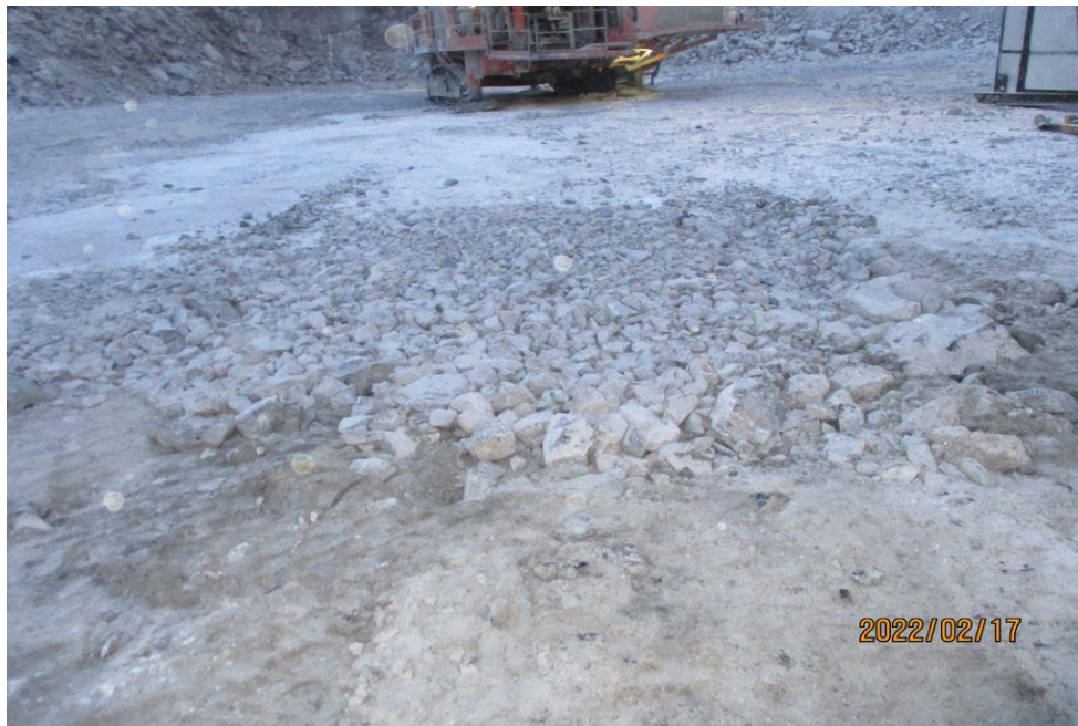
Photo 1. Photo of cleaned up diesel fuel where Shovel 2570 was located during the spill. Note, no visible hydrocarbon staining.
