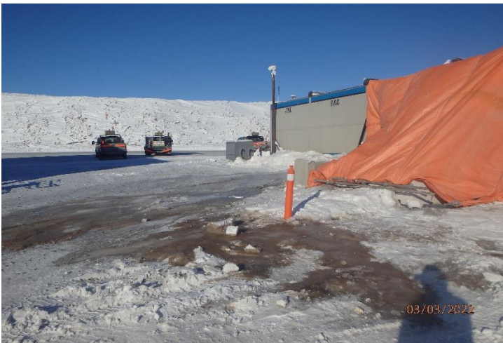
Photo 3: View of frozen sewage from the secondary spill. Photo facing north.
