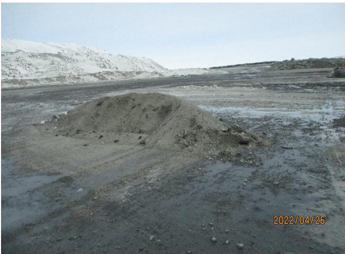
Photo 1: Sable Down Line – View of impacted material piled up in preparation for loading and hauling to the Land Farm.
