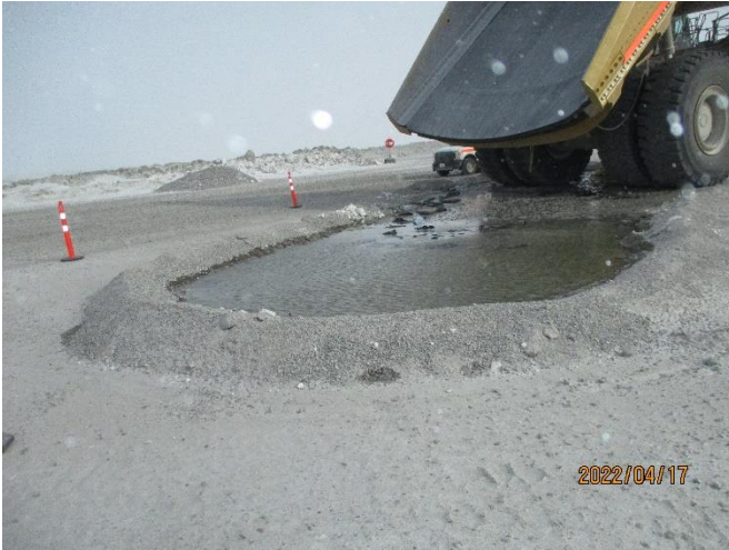
Photo 1: Sable Truck Park Area – View of small berm containing fuel. Note that the spill occurred on compacted/flat ground.
