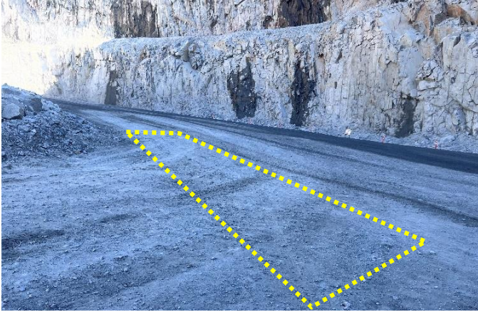
Photo 1: Sable Pit Ramp – View of area where hydraulic oil spilled from Shovel 2570 (highlighted in yellow).
