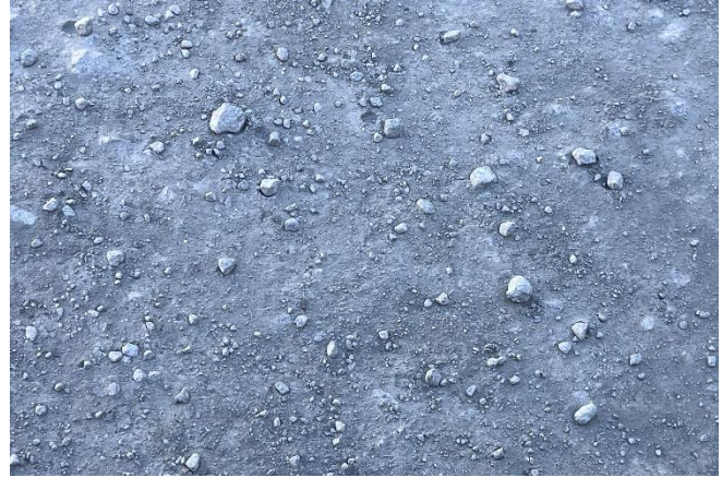
Photo 2: Sable Pit Ramp – Close-up view of bare rock portion of the pit ramp.
