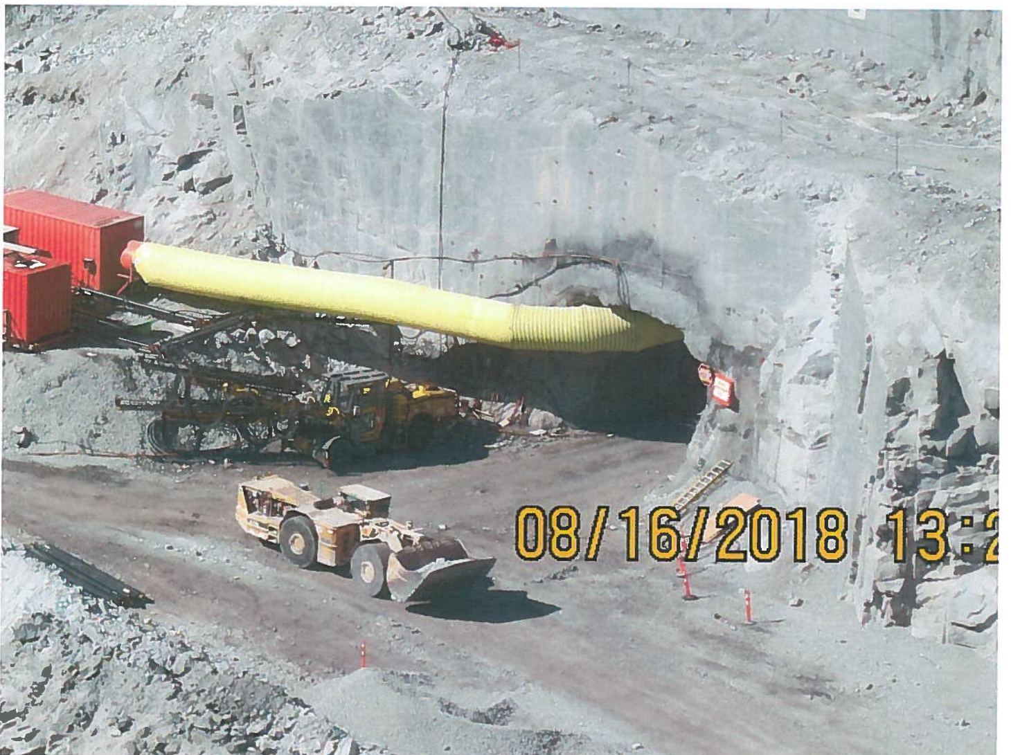
Photo 12: 2235 Portal - A scoop tram is used to remove the waste blast rock. The PAG free waste rock is currently being used for the catch berms on the road. Rock is also being disposed of off the existing ramp road.
