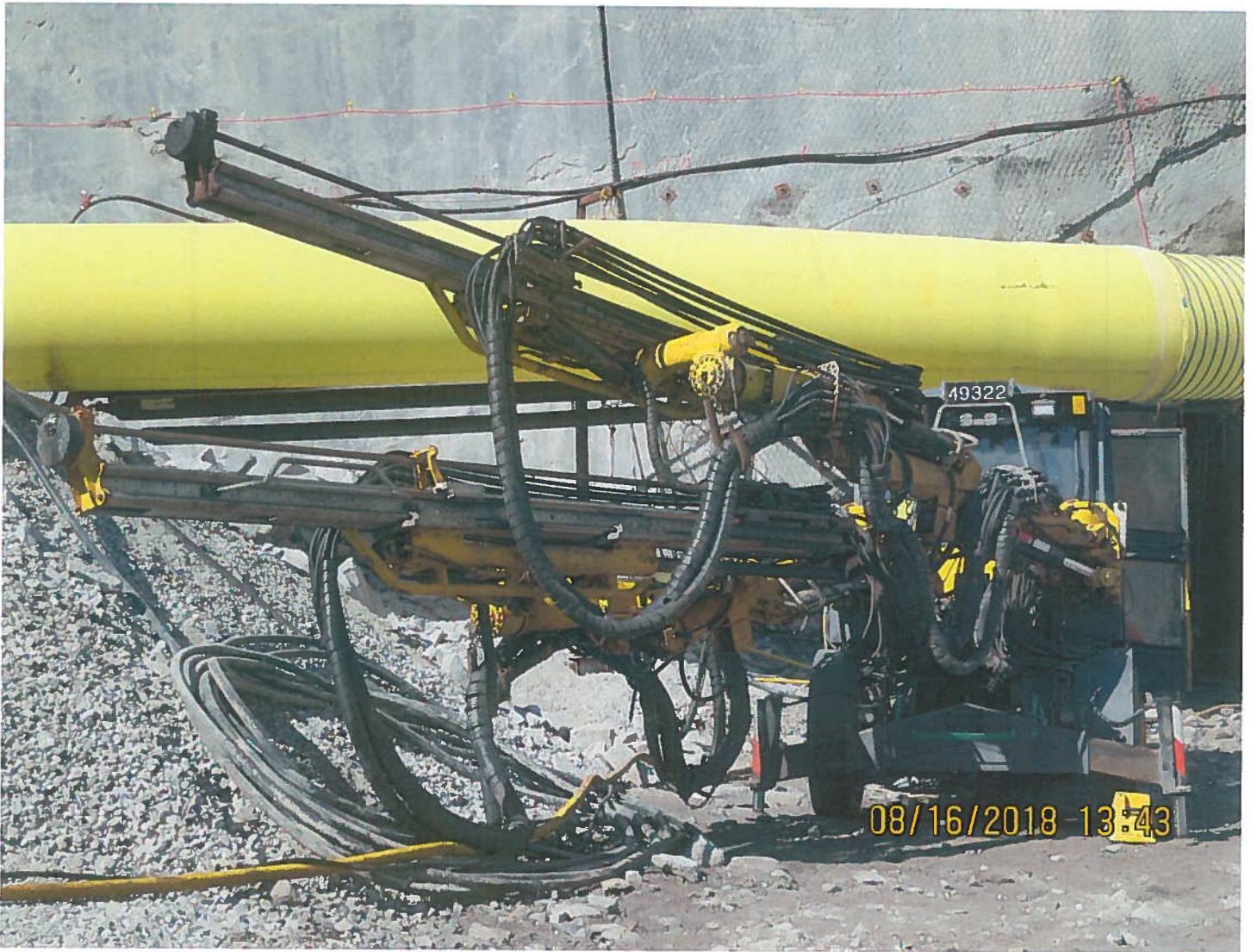
Photo 11: 2235 Portal - An Electric Drill that is being used for Portal advancement.
