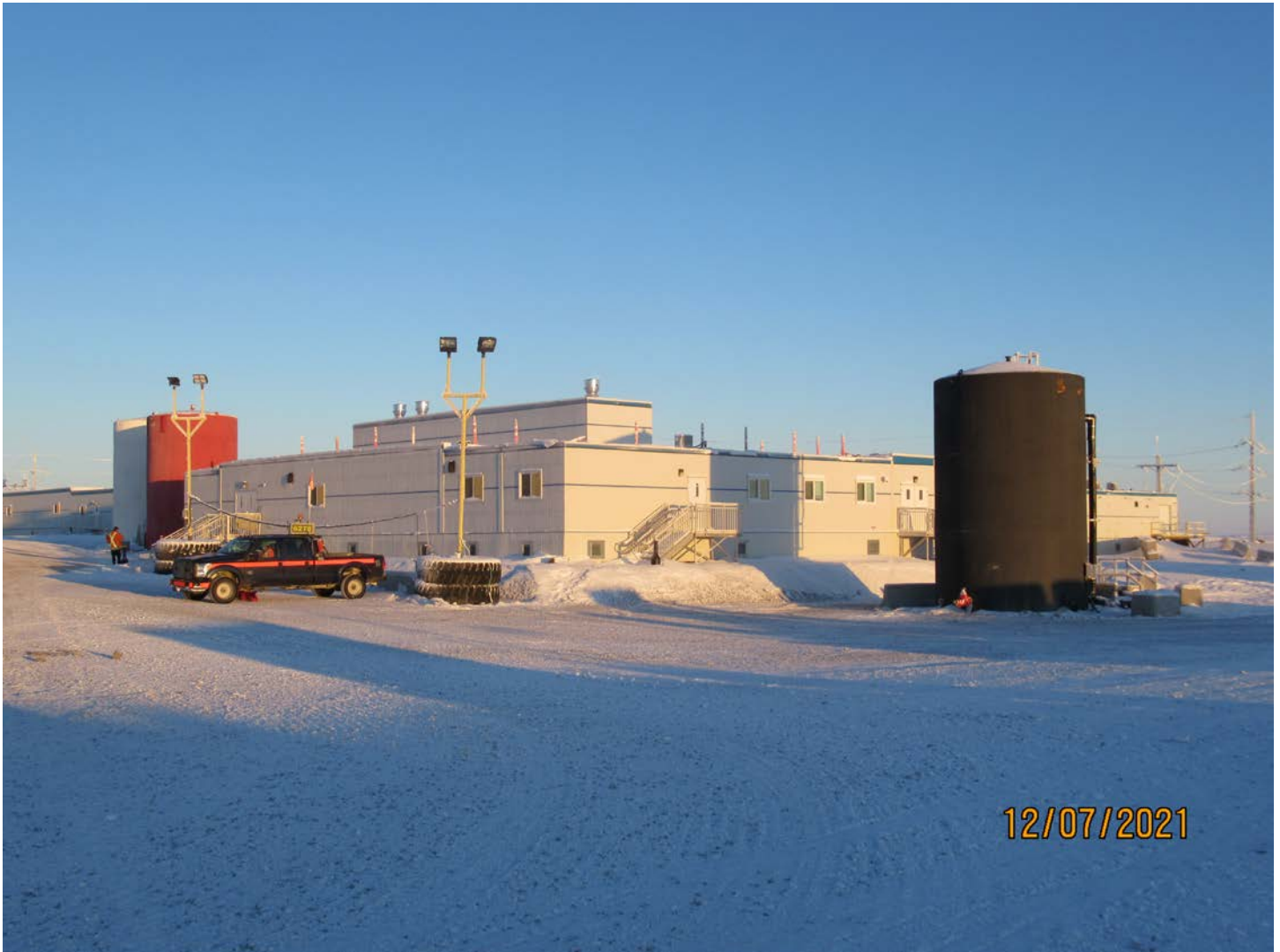
Photo 37: The Misery Camp parking area. The white tank holds potable water, the red tank contains fire suppression water and the camp sewage reports to the black tank on the right.
