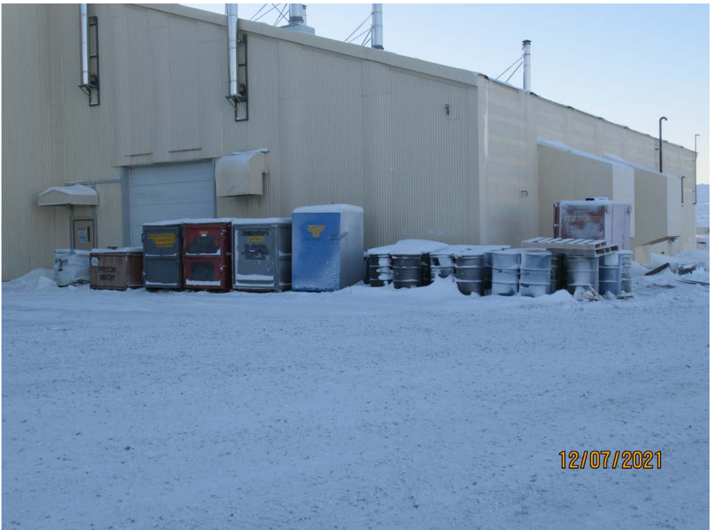
Photo 34: The waste station at the Misery Camp truckshop.
