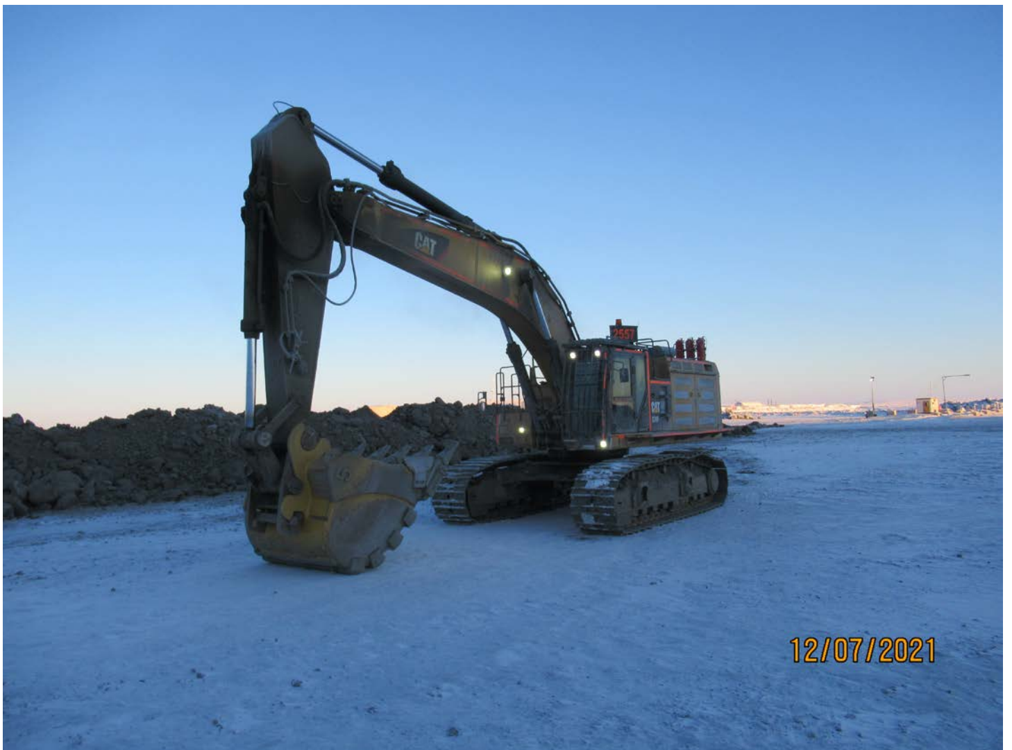
Photo 8: This excavator is used to sort and pile the ore at the laydown in Photo #7.
