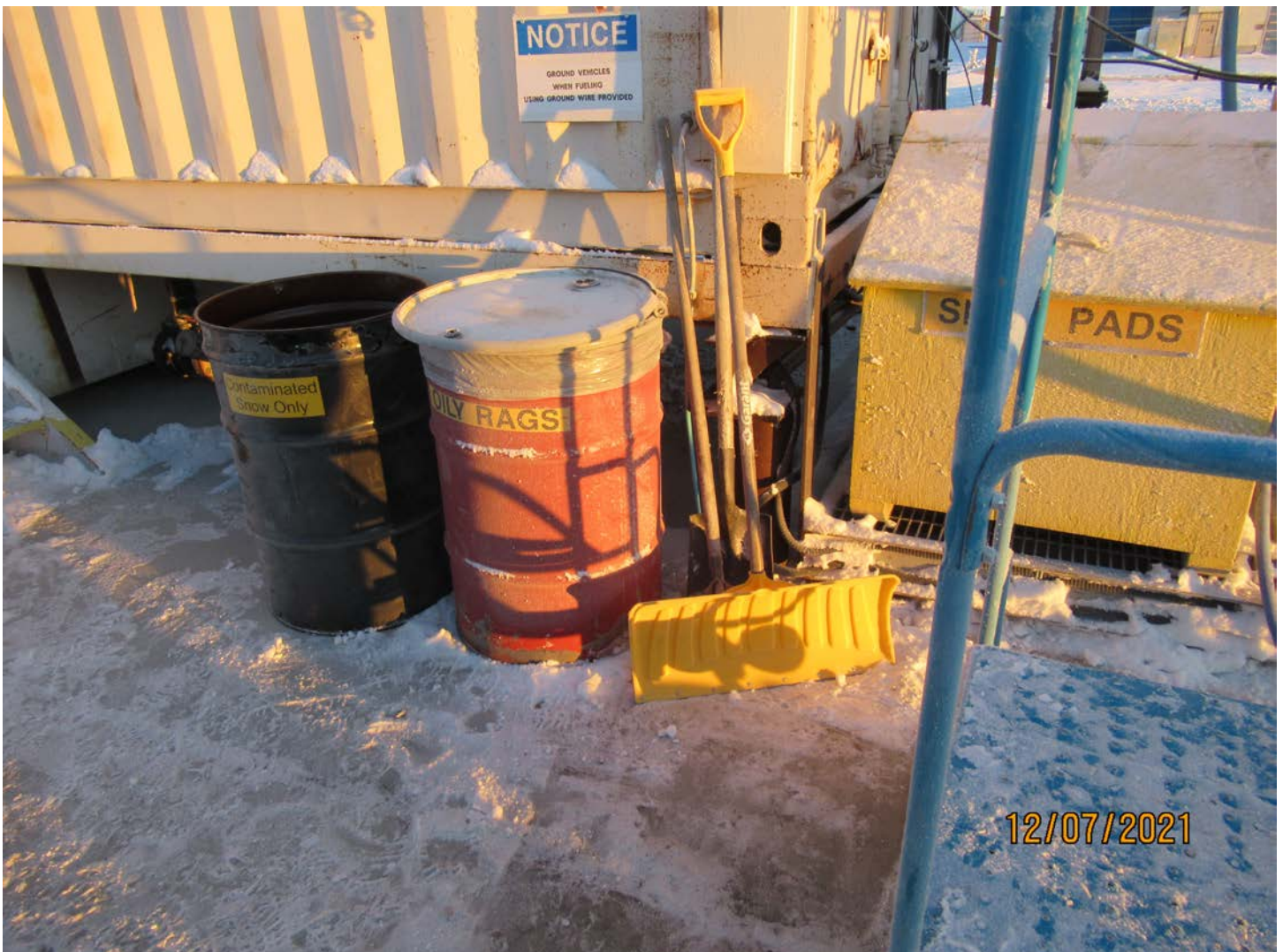
Photo 22: Hydrocarbon impacted waste is being placed in designated waste containers at the fueling ramp.
