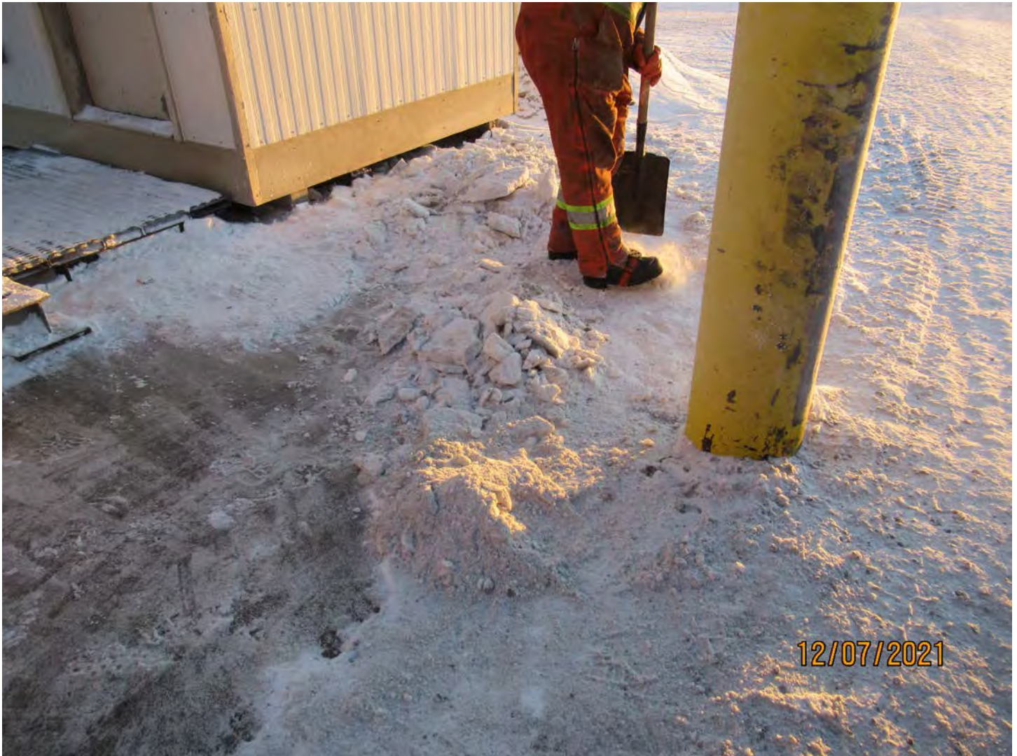
Photo 21: A mine employee was scraping up hydrocarbon impacted snow at the light vehicle fueling area.
