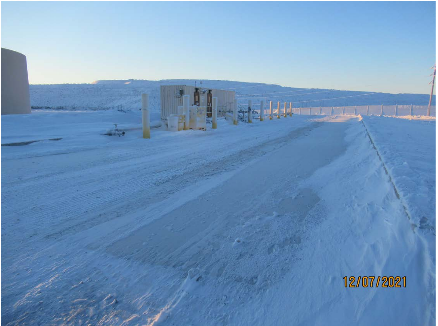
Photo 17: As seen, the snow was cleared from the bulk fuel offload ramp and there were readily available spill response materials staged on the ramp.
