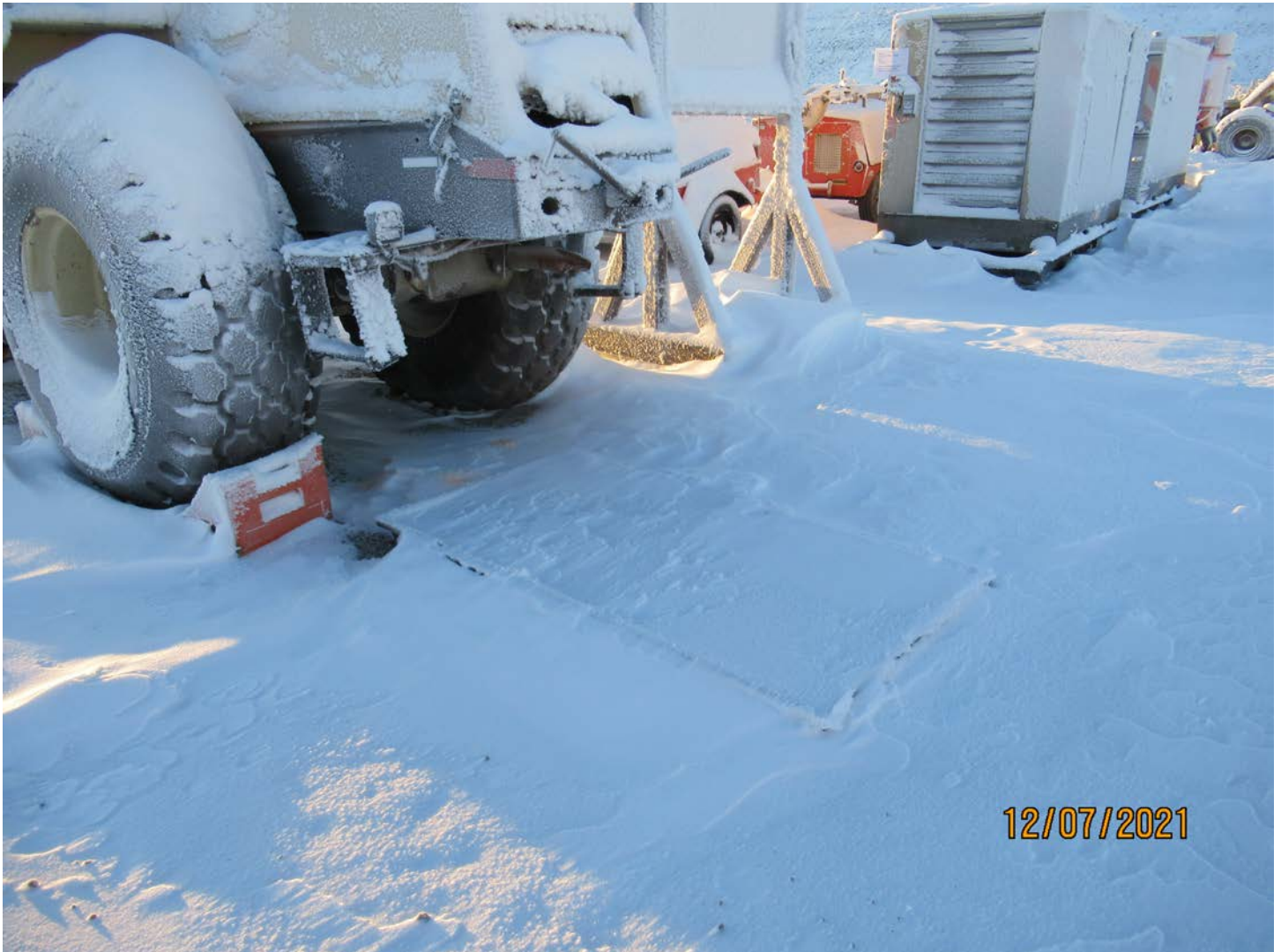
Photo 25: As seen, the secondary containment under this equipment was filled with snow and required maintenance.
