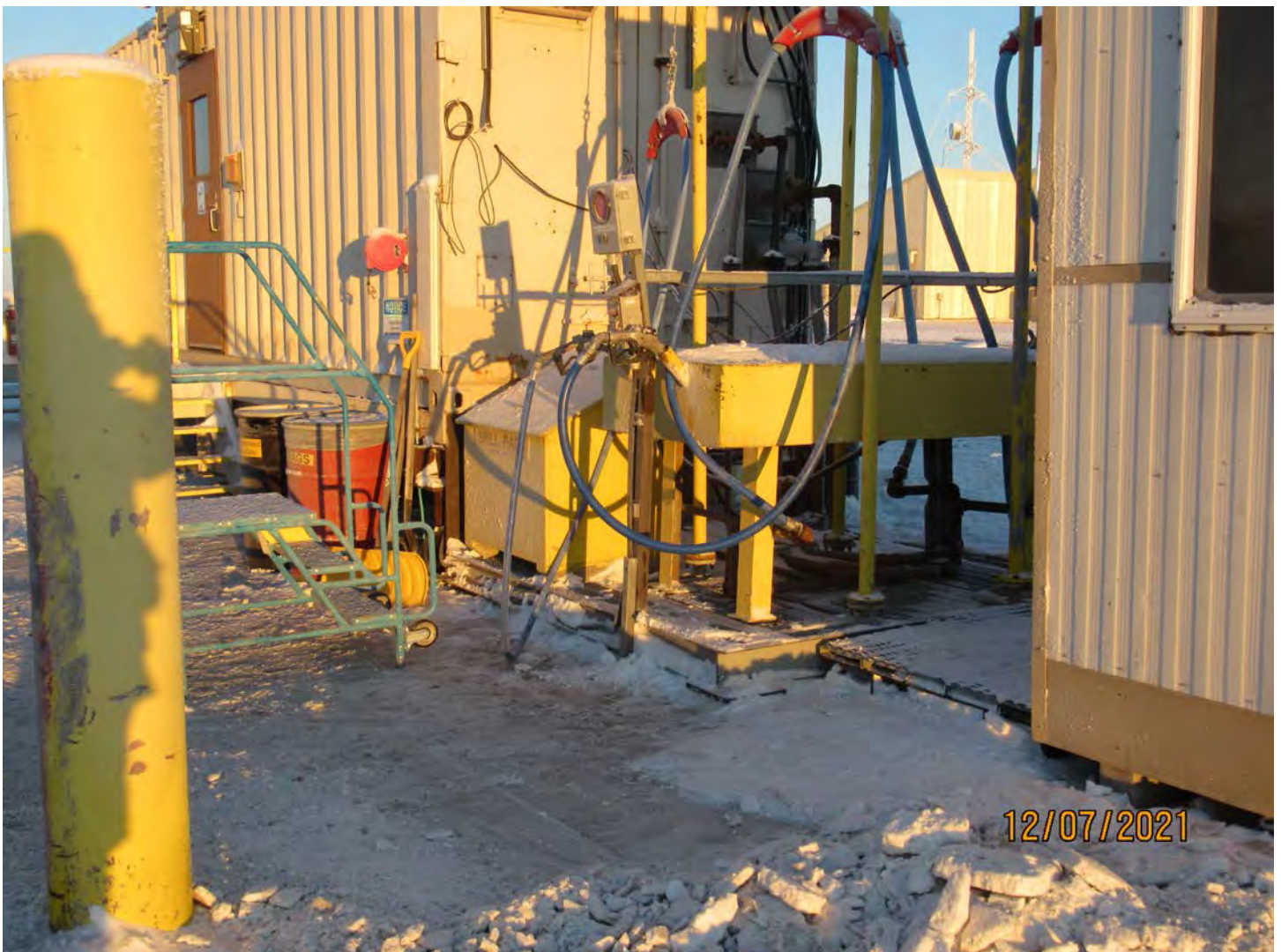
Photo 20: There was secondary containment for the fuel nozzles on the ramp and readily available spill response materials.
