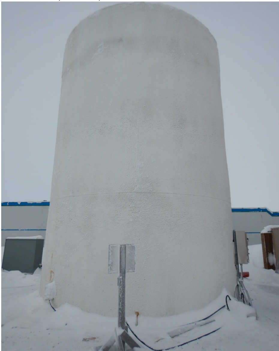
Photo 2 – Misery surface – potable water tank
