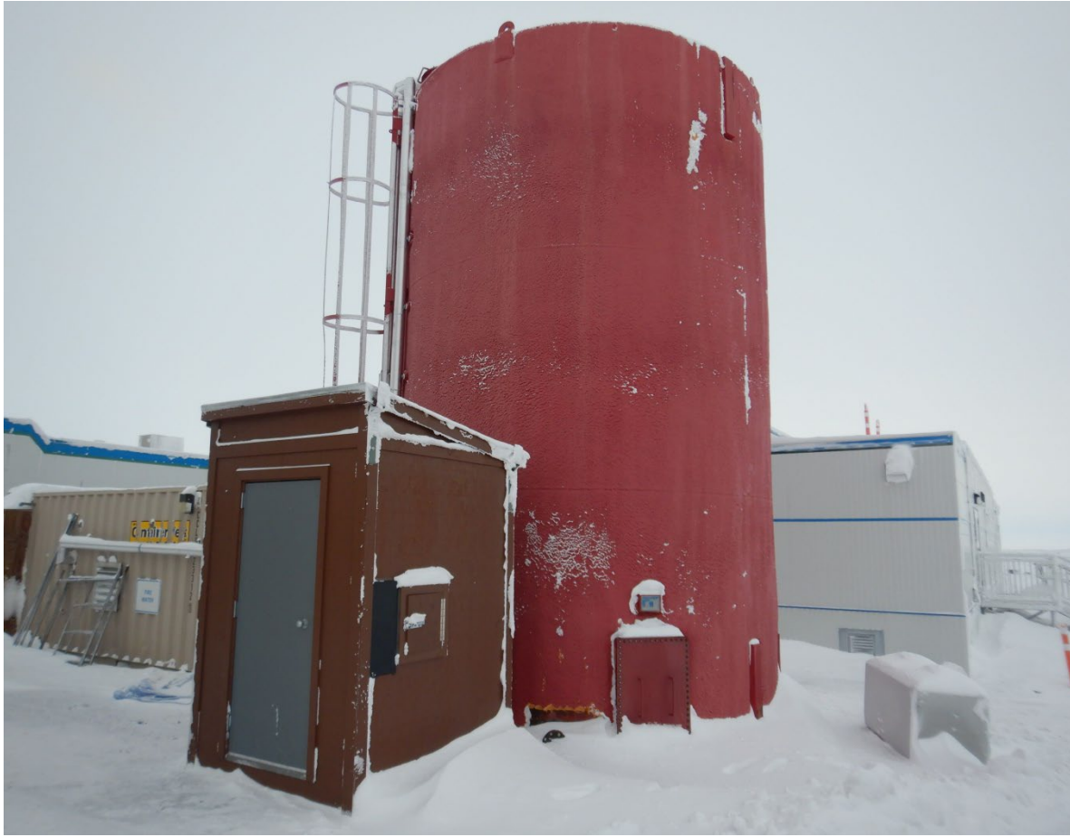
Photo 1 – Misery surface – fire suppression water tank.
