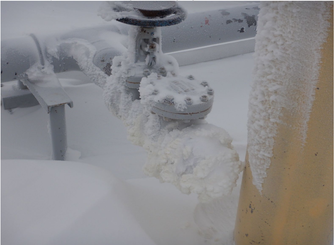
Photo 11 – Misery surface – Diesel fuel storage area – Leaking flange.
