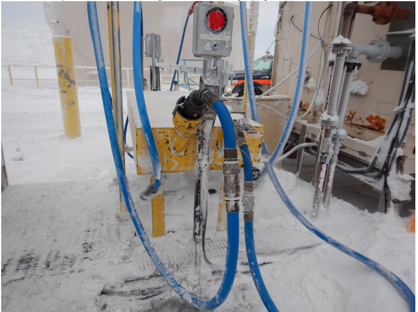
Photo 14 – Misery surface – Diesel fuel storage area – Snow clearing in progress (2).
