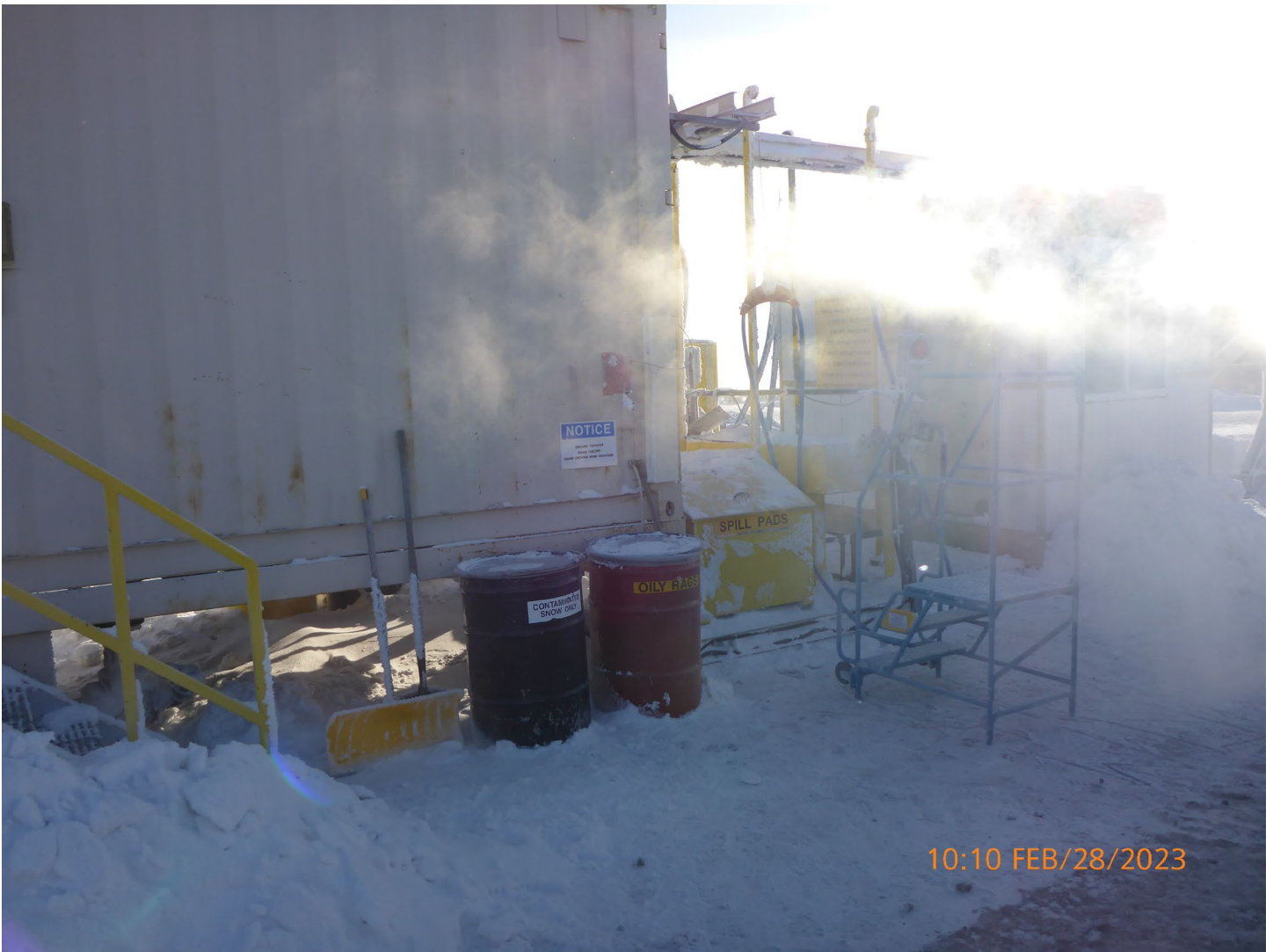
Photo 1 – Misery Refueling Station – Refueling station was clean and well organized. Waste containers were labelled and there was no indication of misdirected waste.
