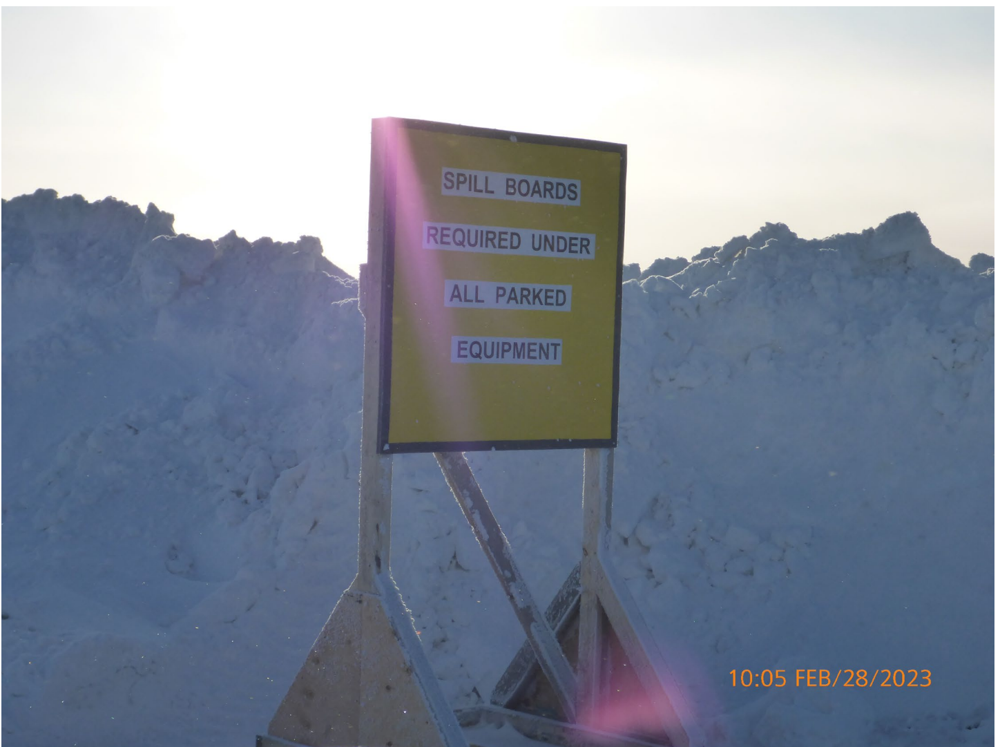
Photo 10 – Drip Trays – A campaign at the misery camp has been initiated to ensure that all parked equipment deploys drip trays as per Condition 37 of the Land Use Permit.
