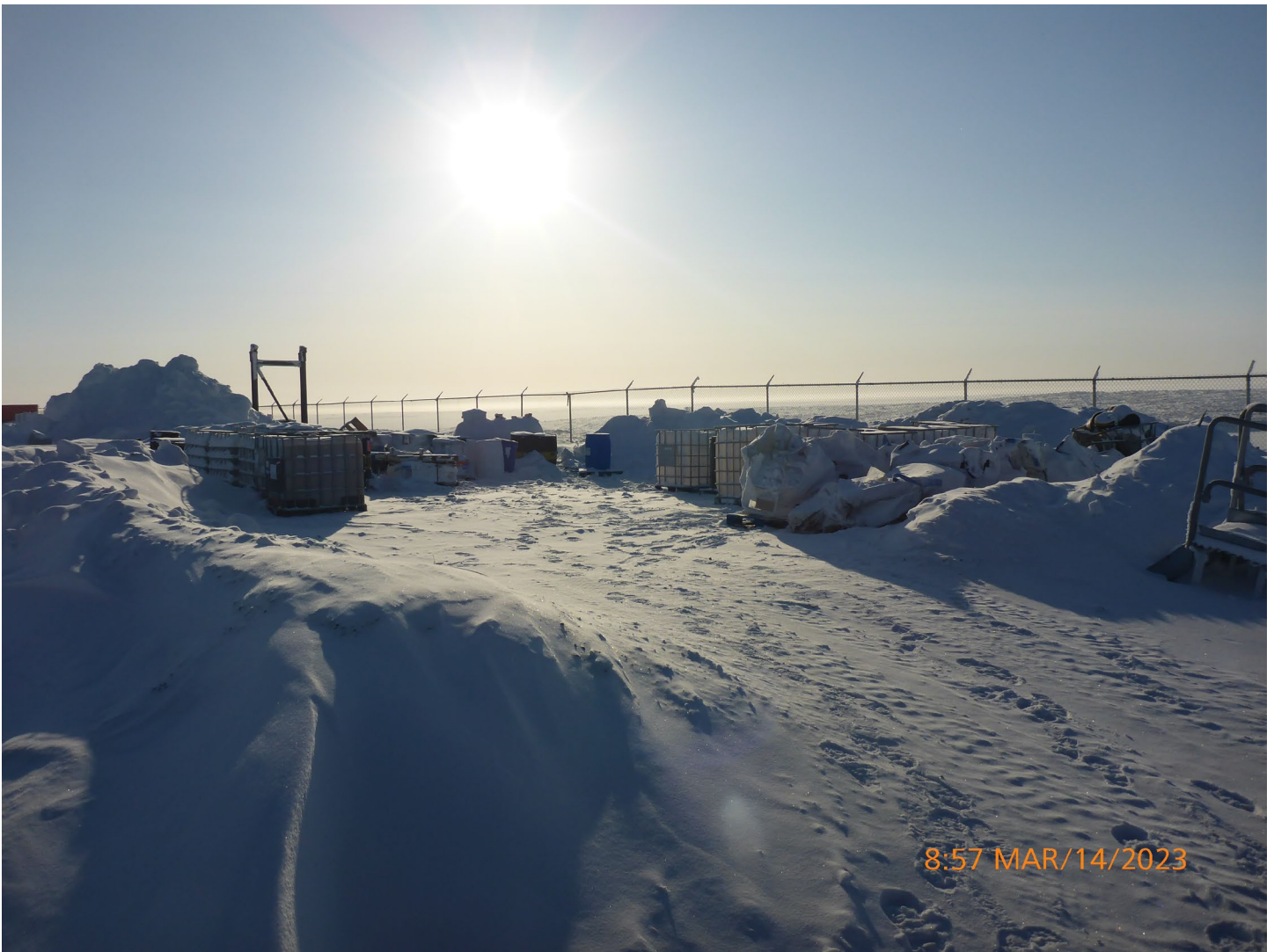
Photo 13 – Misery Hydrocarbon Storage – The hydrocarbon storage area is a lined facility used to store hydrocarbon and other potentially hazardous materials. Several of the containers required labels, and many of the containers have been in the area for an extended period. The Inspector recommends that Arctic go through the area and review which containers are no longer needed and remove from site.
