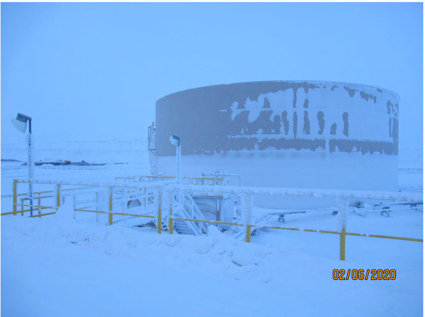
Photo 20: The main fuel storage facility at Misery Camp.
