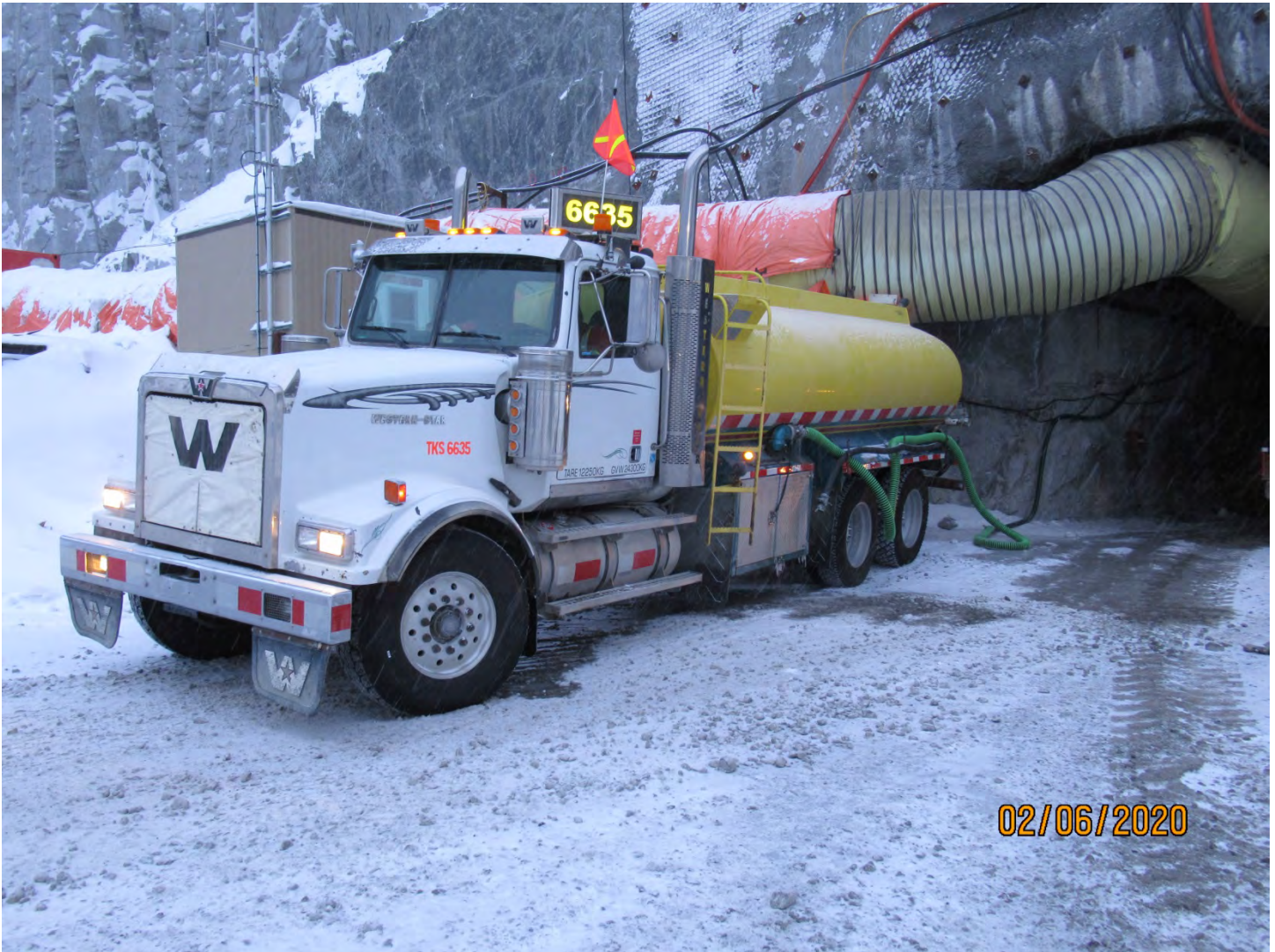
Photo 5: Trucked water was being pumped into the UG water system in support of the UG mining operations.
