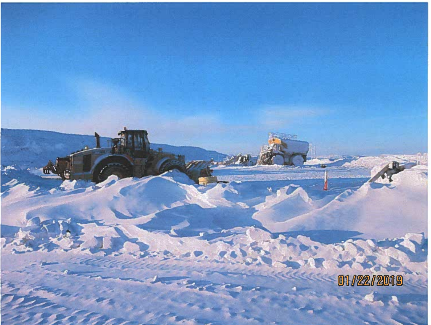
Photo #28 - W2017D0004 Crews were repairing equipment in the camp equipment laydown.
