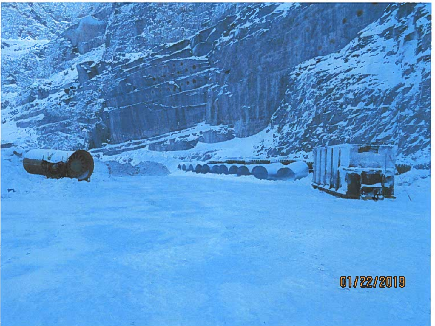
Photo #2 - W2017D0004 Materials including a waste bin and fresh air tubing for the underground staged at the switchback laydown.
