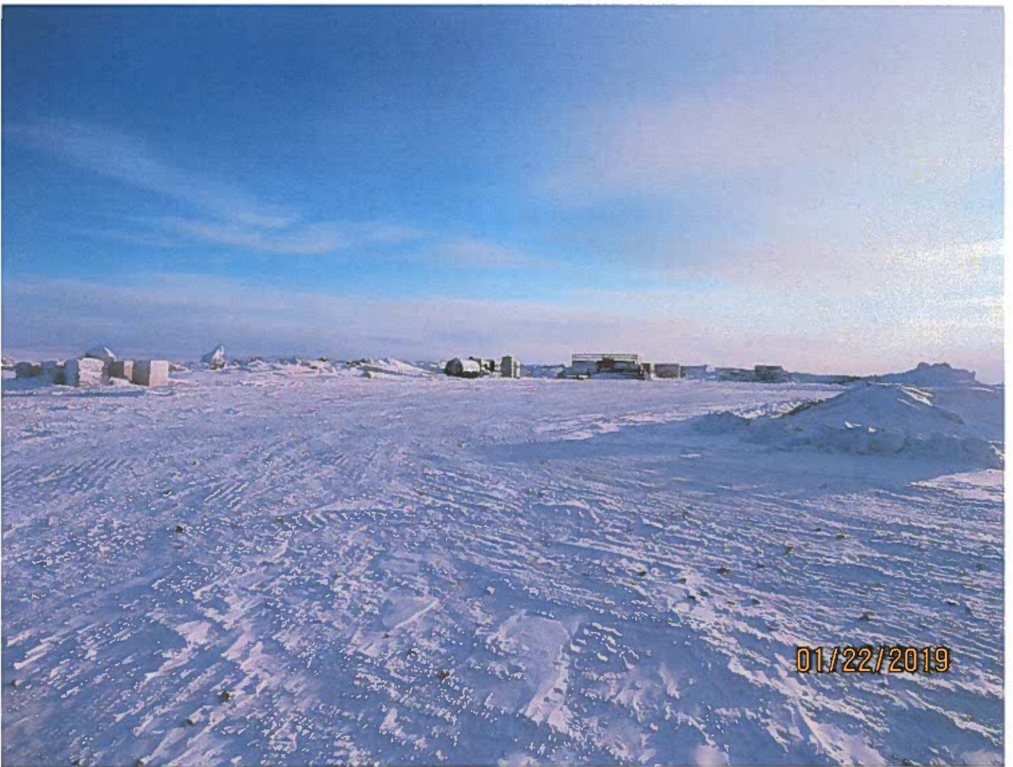
Photo #29 - W2017D0004 The laydown at the top of the Misery Pit ramp appeared ready to receive materials.
