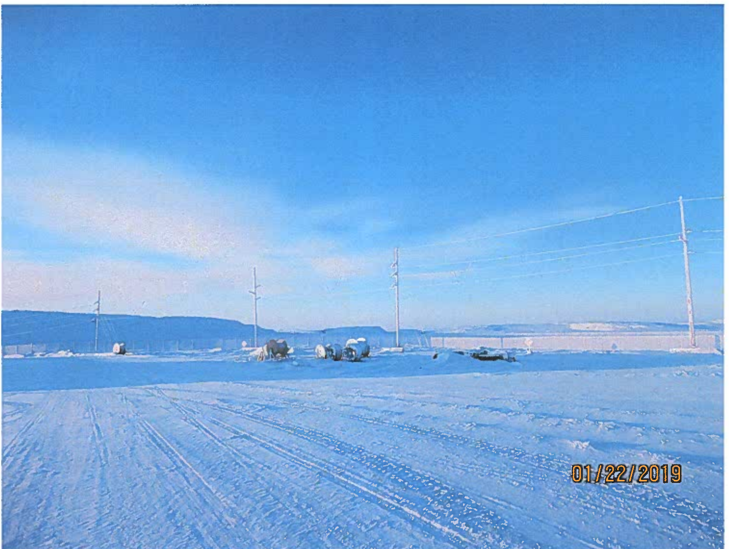
Photo #26 - W2017D0004 This laydown adjacent to the camp fuel storage facility is ready to receive materials transported along the winter road.
