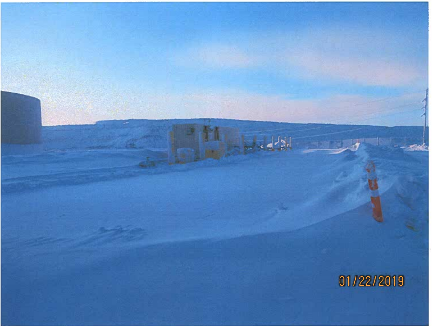
Photo #35 - W2017D0004 This transfer station is used to offload fuel brought to site during the winter road season.
