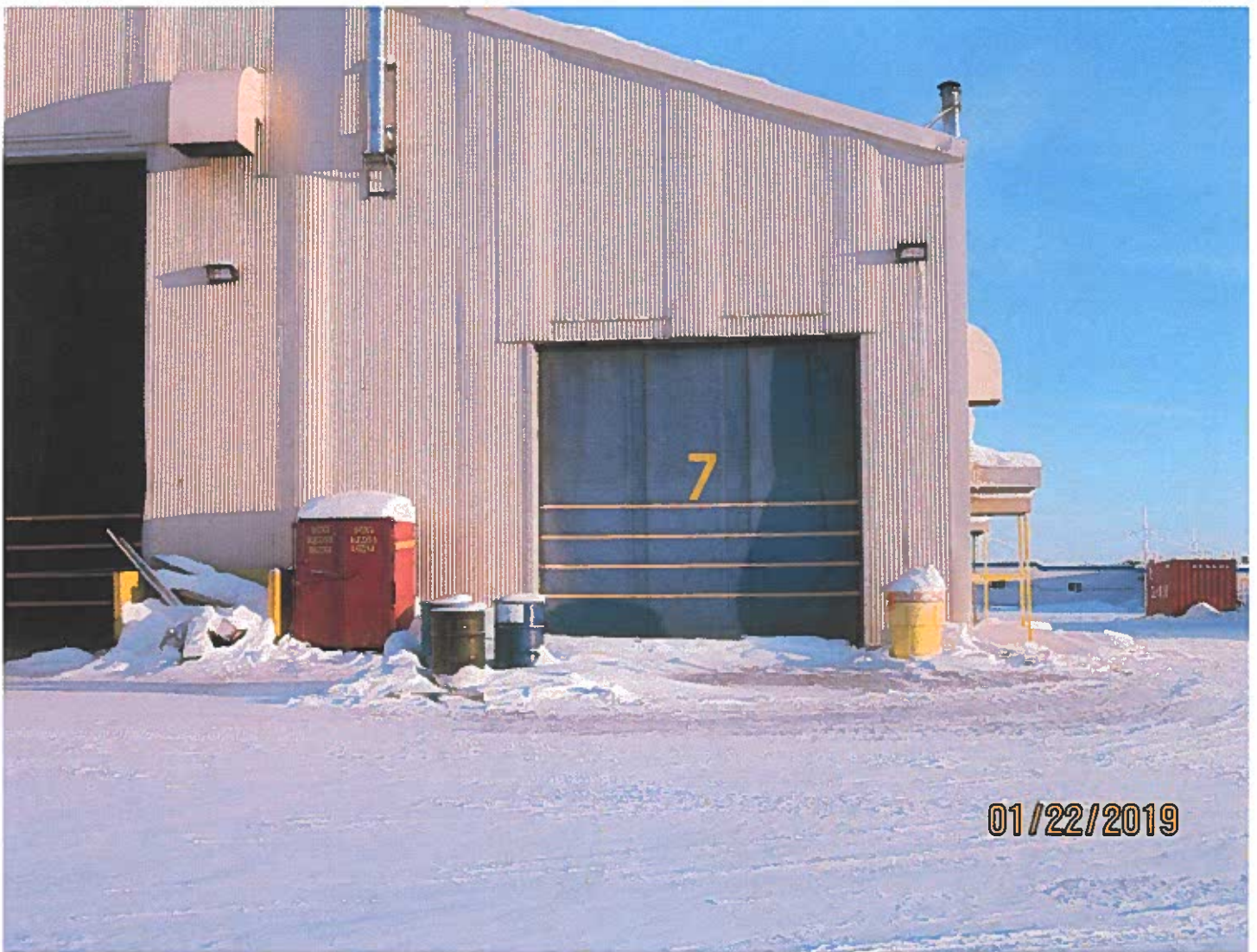
Photo #25 - W2017D0004 An example of properly segregated, staged & labeled waste and a spill kit at Misery Camp.
