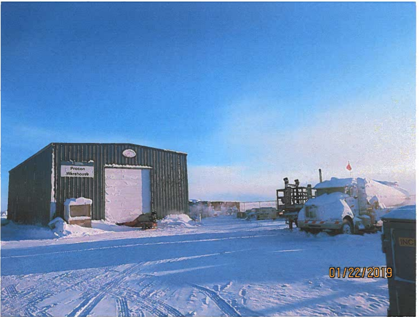
Photo #23 - W2017D0004 The Misery Camp Cold Storage Building.
