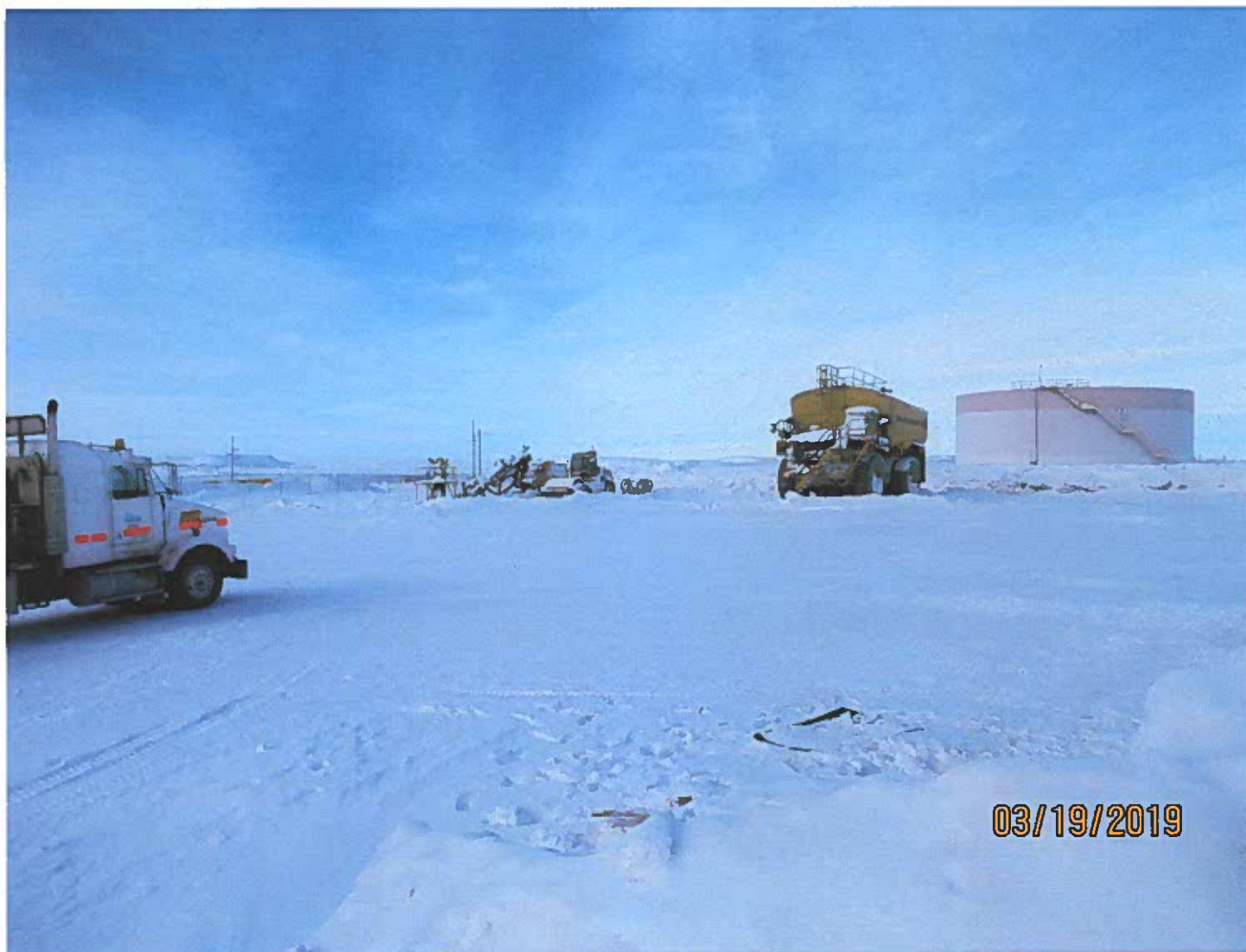
Photo #23 - W2017D0004 MUG Project The heavy equipment laydown at the Misery Camp.
