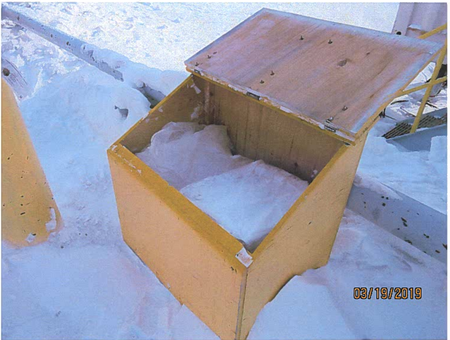
Photo #15 - W2017D0004 MUG Project There were readily available spill response materials at the bulk fuel transfer facility.
