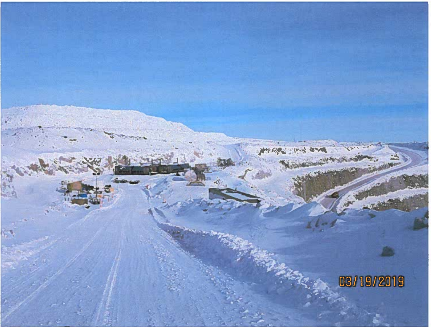
Photo #1 - W2017D0004 MUG Project A look at the infrastructure along the 440 Bench that will be used for the underground operations.
