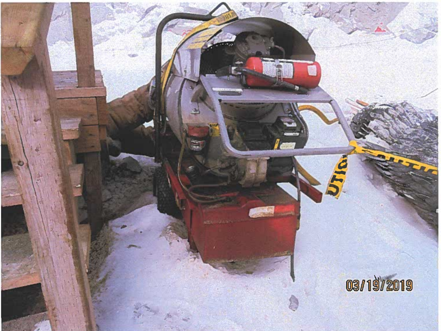
Photo #10 - W2017D0004 MUG Project
